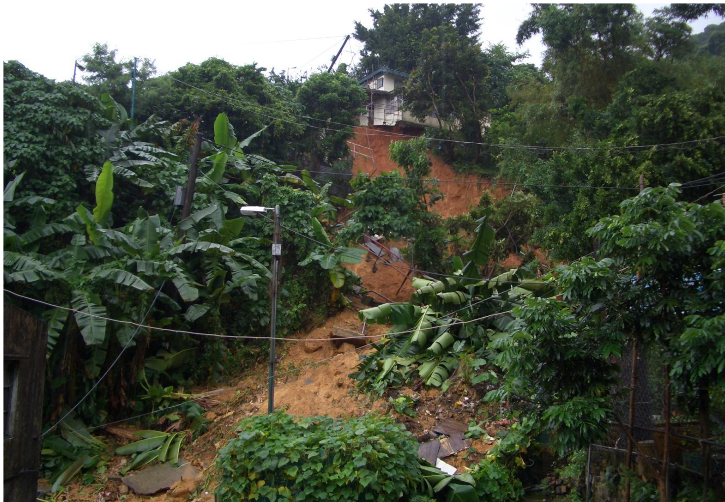
Plate 2 - Front View of the 20 August 2005 Landslide (Photograph taken on 21 August 2005)
