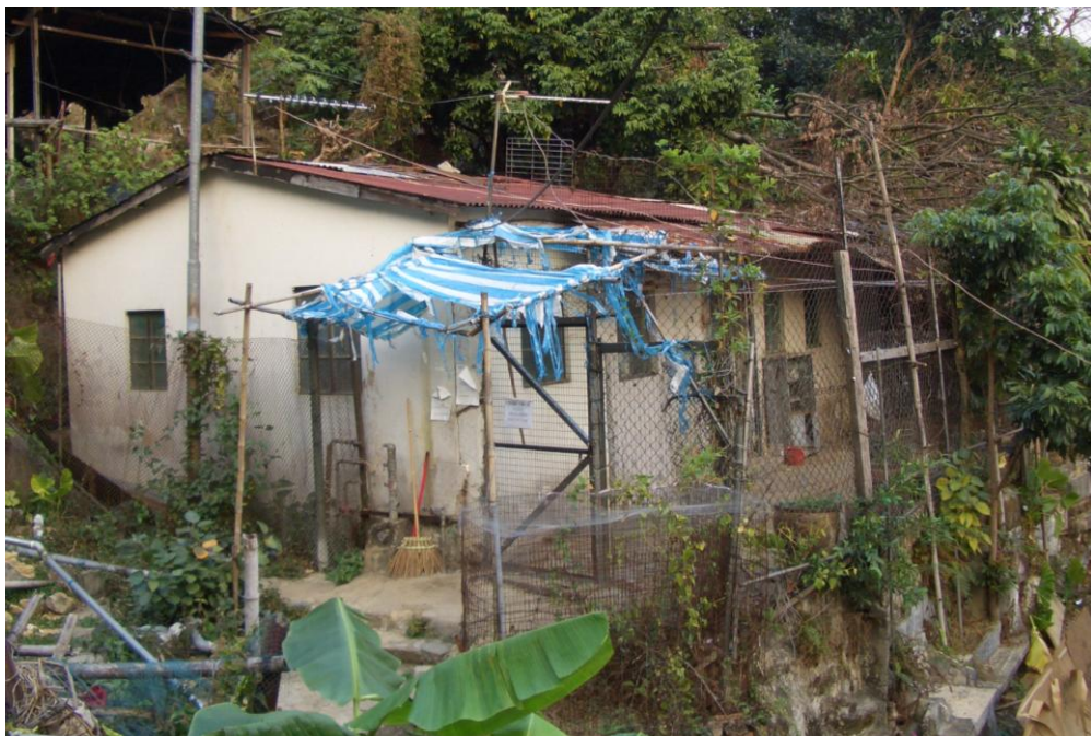
Plate 9 - Registered Squatter Structure No. RTW/4A/526 (Photograph taken on 5 December 2005)
