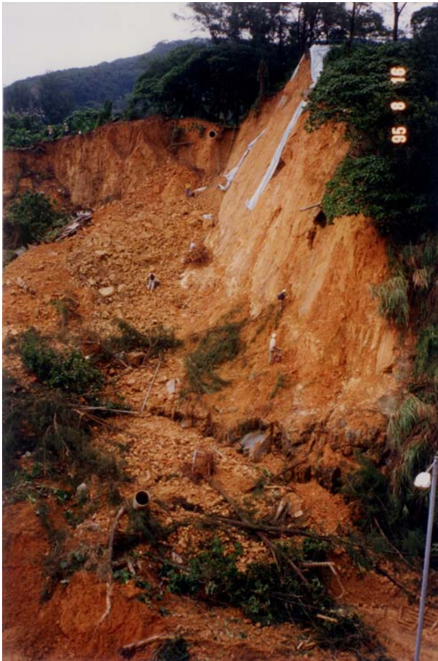
Plate 8 - Weathered Rock Joints Forming the Back Scarp of the Landslide (Photograph Taken on 19 August 1995. See Figure 21 for Location)
