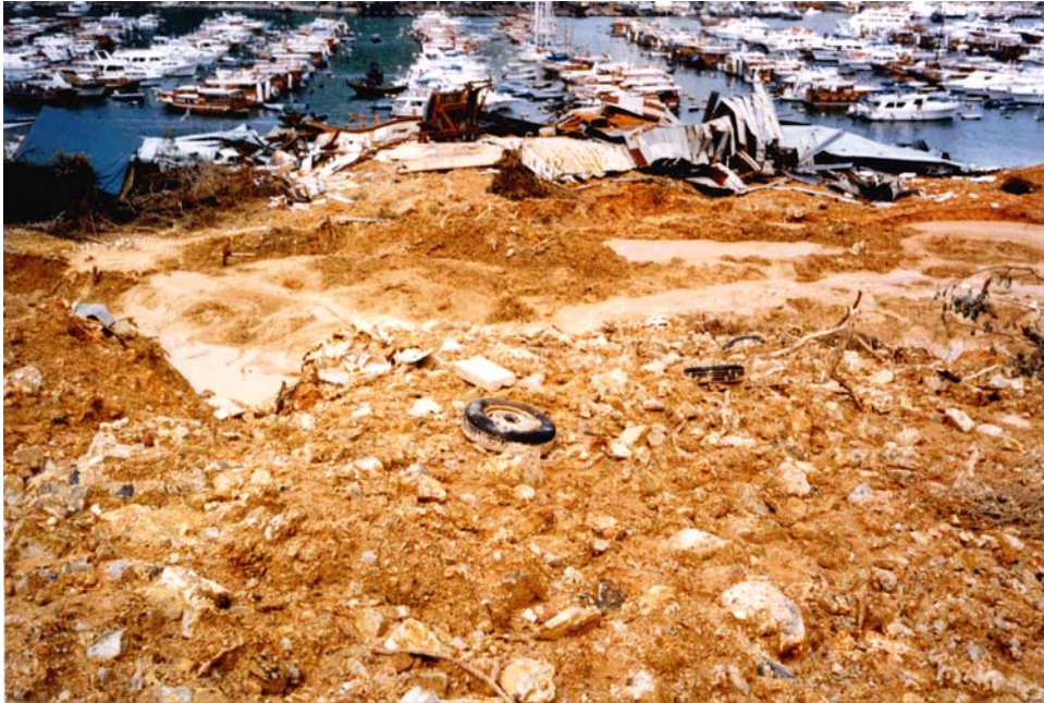
Plate 4 - Debris with Fill Material and Refuse on Landslide Scar
