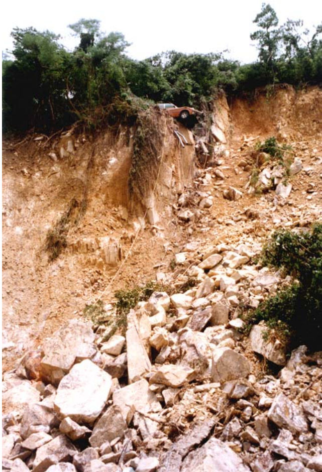
Plate 7 - Rock Debris on Landslide Scar
