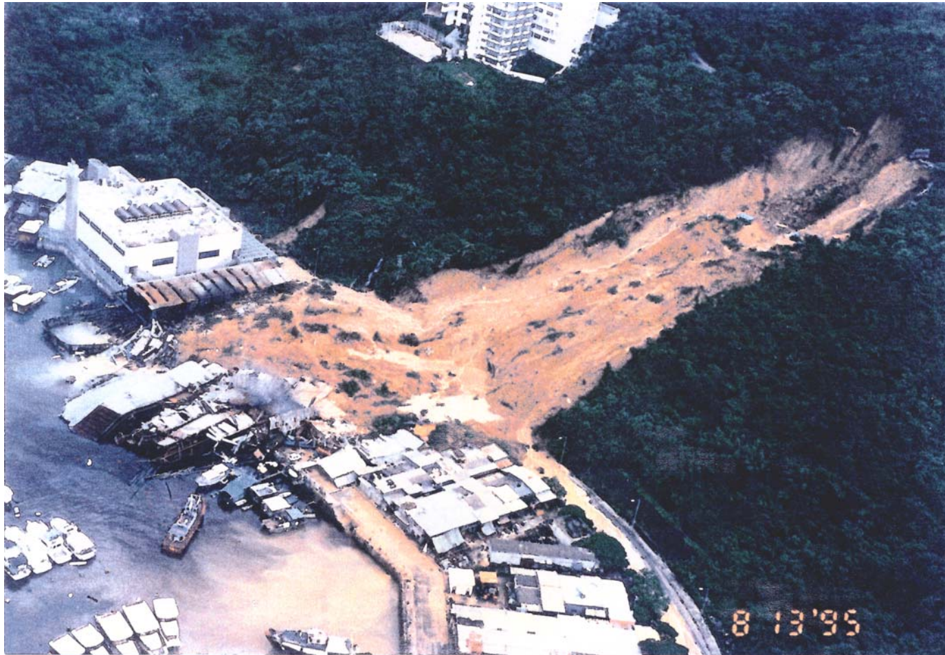
Plate 1 - The Landslide on 13 August 1995
