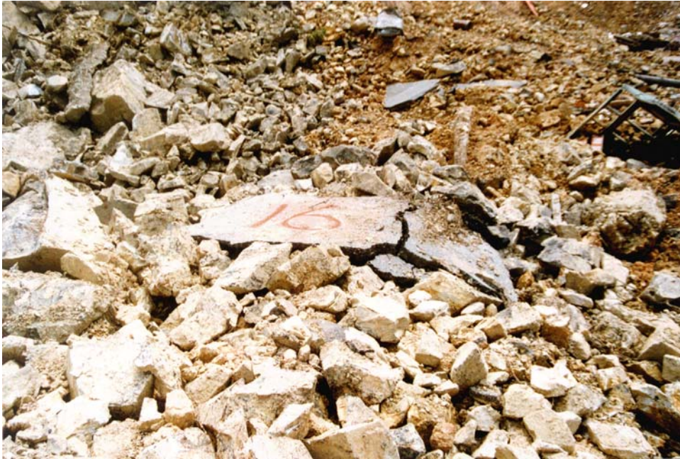
Plate 6 - Bituminous Pavement (1.5 m x 1 m) on Upper Part of Landslide Scar
