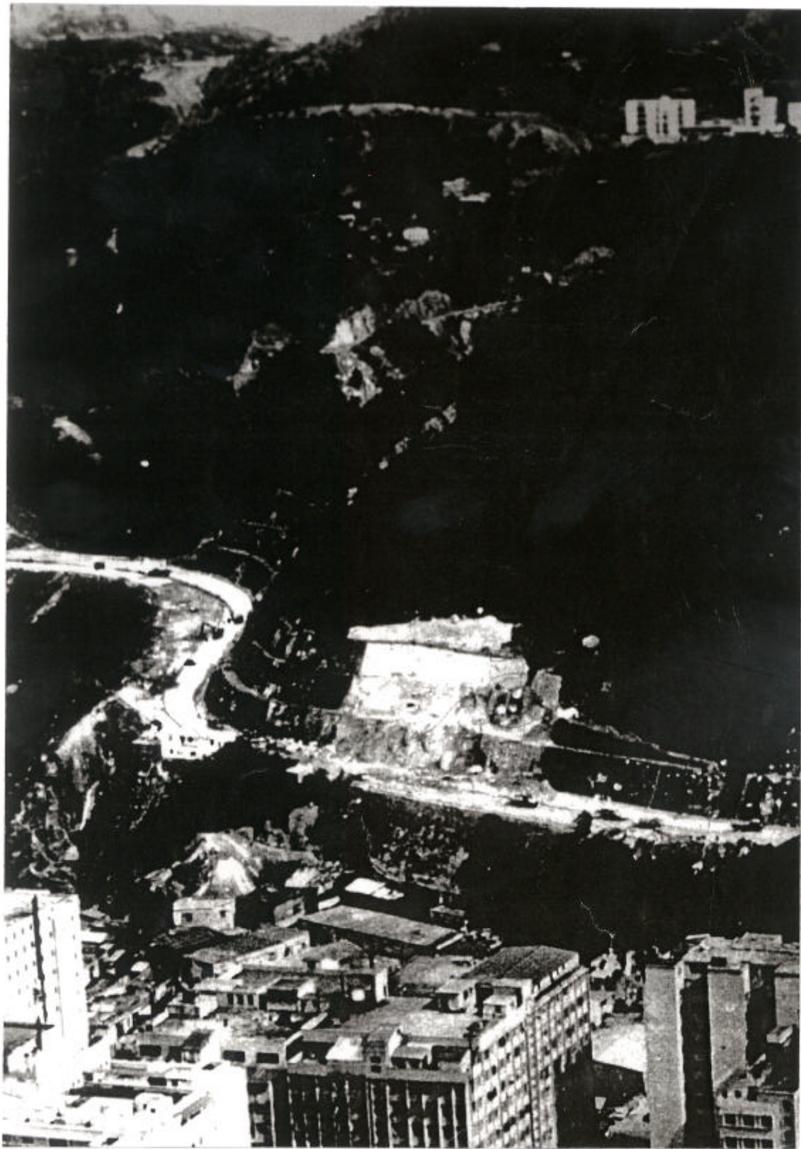
Plate 8 - View of 1972 Failure (Photograph Extracted from Figure 1 of Maunsell, 1972)
