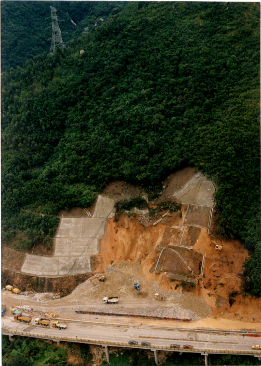
Plate 1 - View of 3 August 1997 Landslide (Photograph Taken on 8 August 1997)
