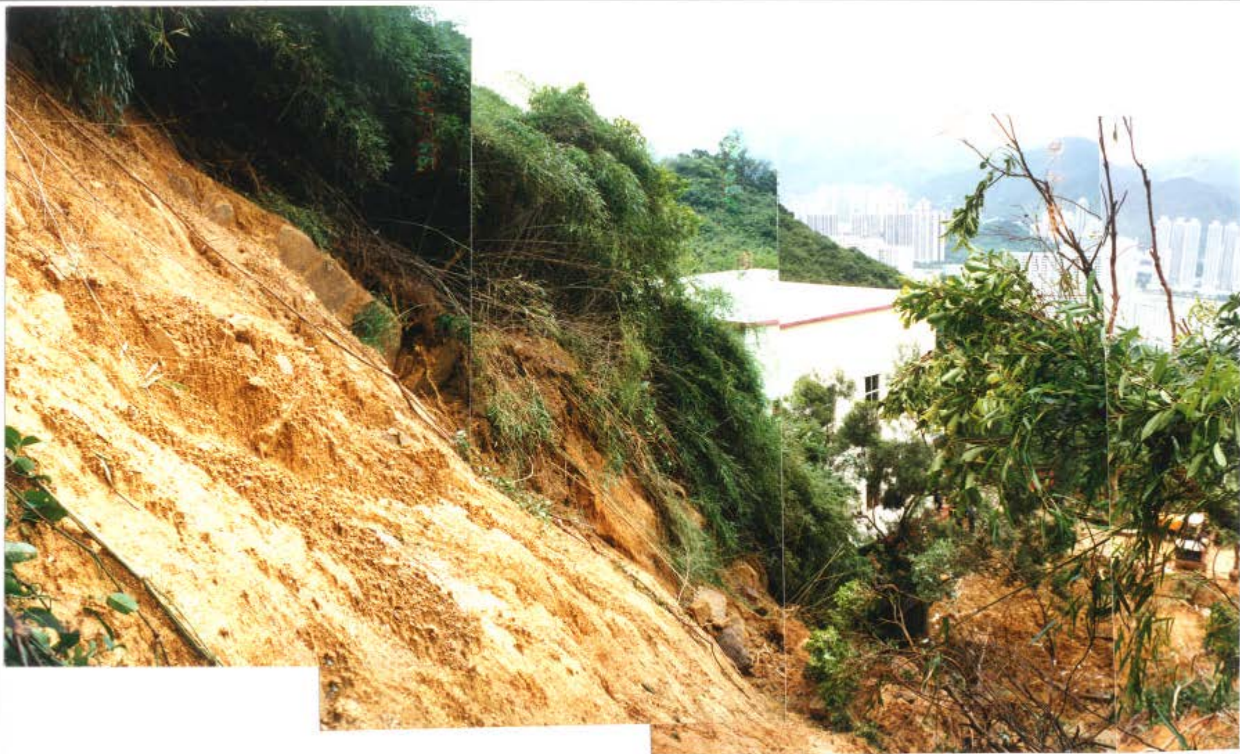
Plate 4 - View of the Sheeting Joint Surface (Photograph Taken on 7 July 1997. See Figure 14 for Location. Note that the Northeast Flank of the Landslide Merges with the Natural Hillside)
