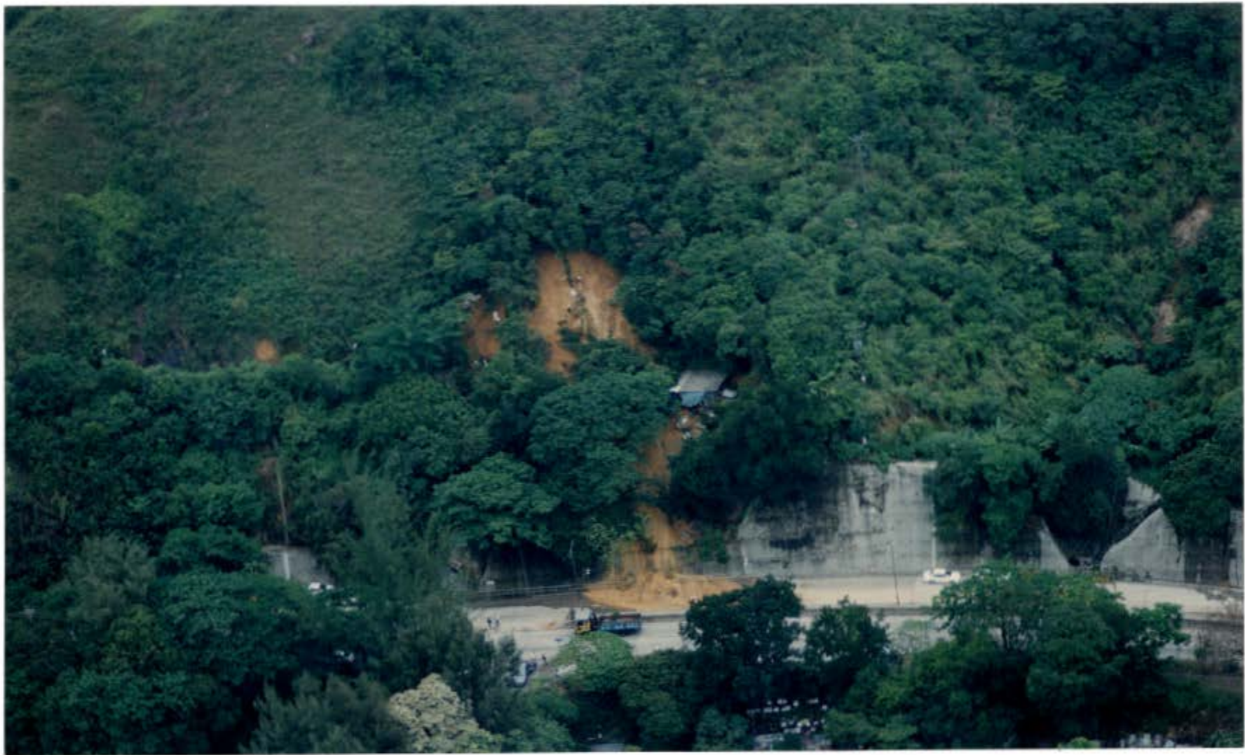
Plate 1 - Photograph of the Site of the Landslides Taken in the Afternoon of 4 June 1997 (See Figure 14 for Location)
