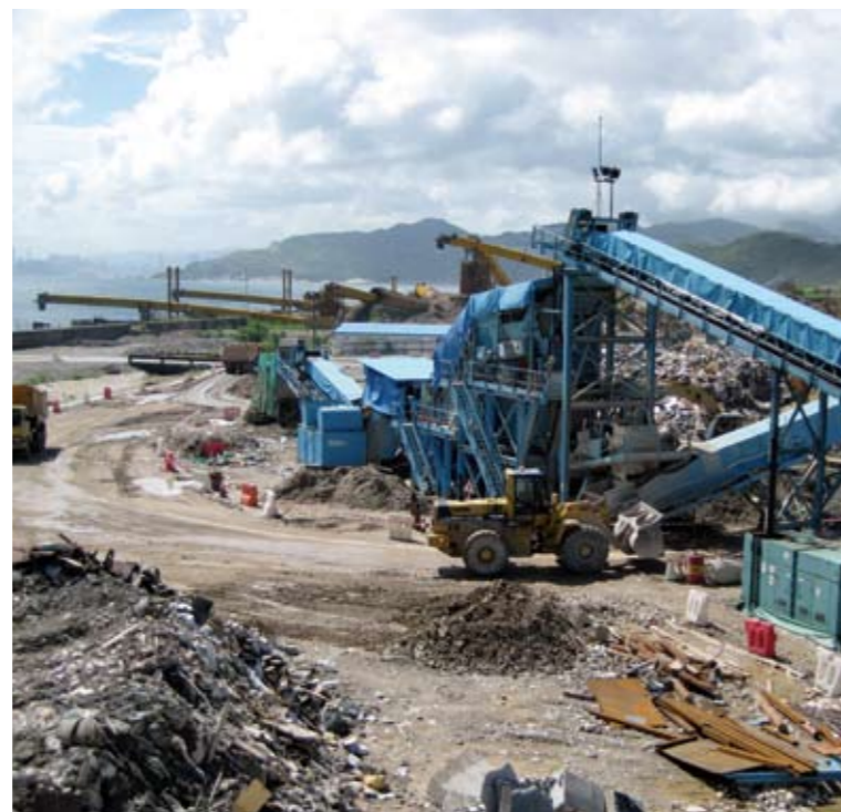
將軍澳第137區的建築廢物處理設施 Construction waste disposal facilities at Tseung Kwan O Area 137
