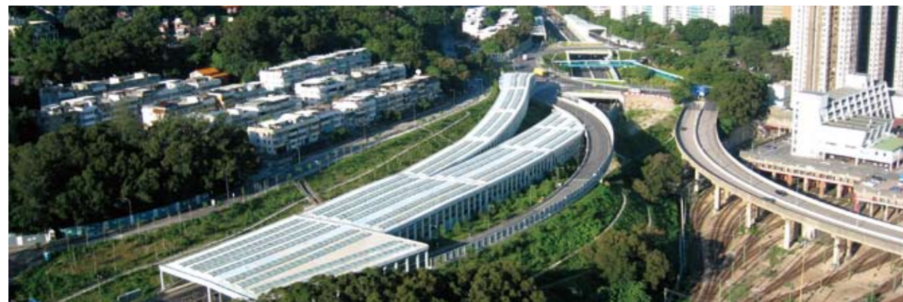
垂直式隔音屏障和半開放式隔音罩 Vertical noise barriers and noise semi-enclosure
