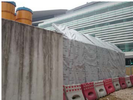
Wan Chai Development Phase II
