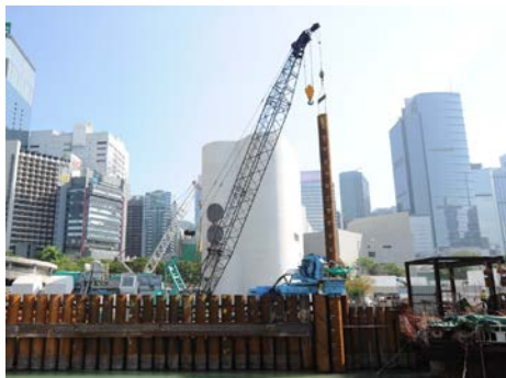
Wan Chai Development Phase II
