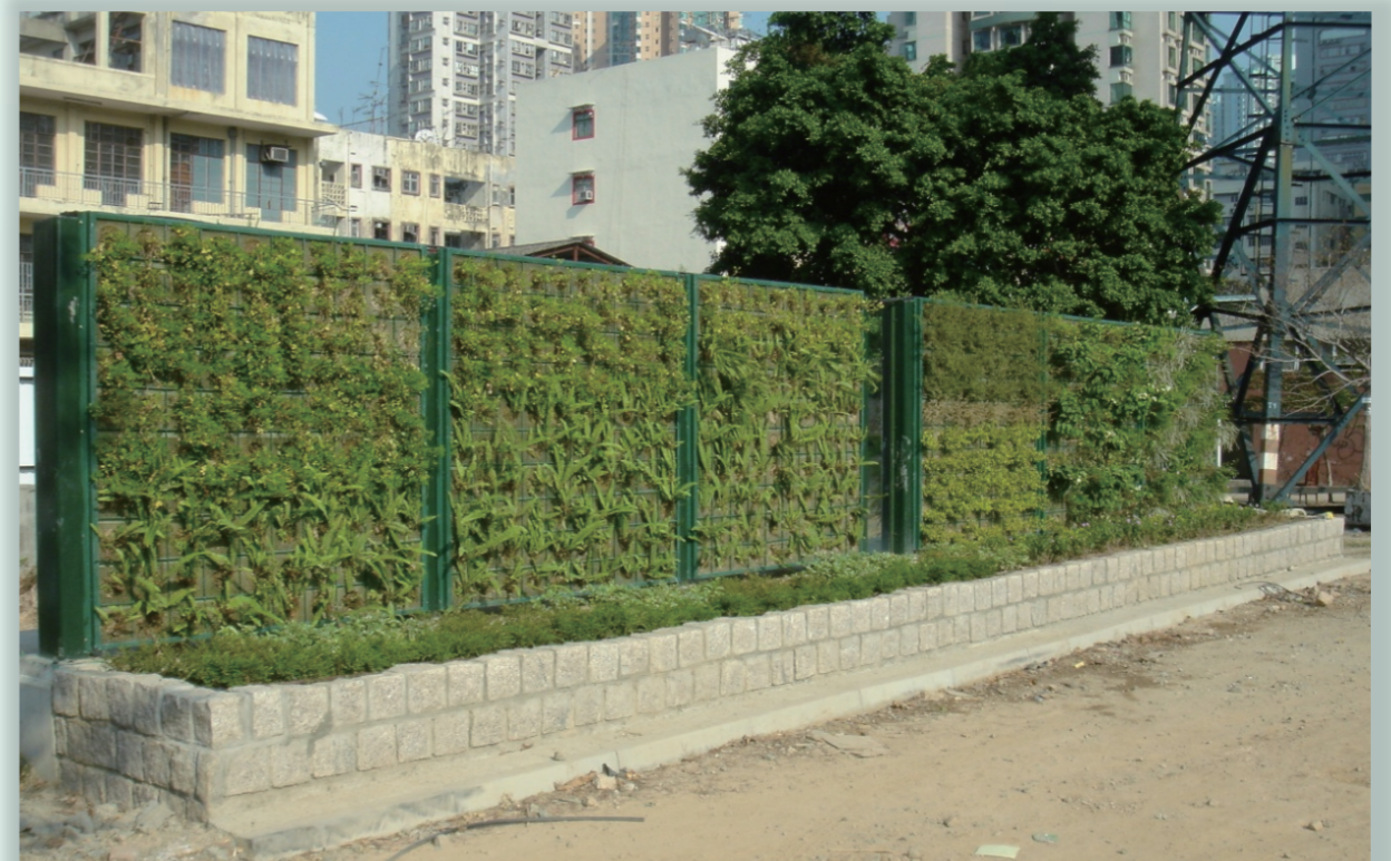
綠化隔音屏障試驗 Trial green wall noise barriers
