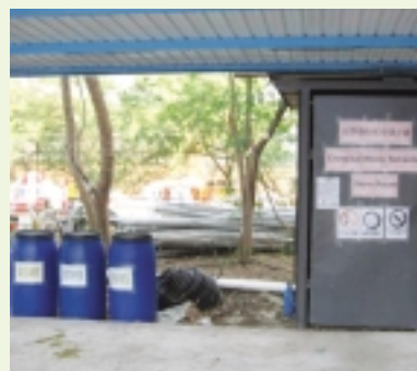
化學廢物臨時貯存設施 Chemical Waste Temporary Storage Facilities
