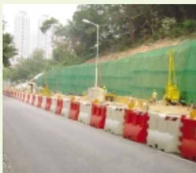
在土坡架設防塵網 Protective netting for suppressing dust emission at soil slope
