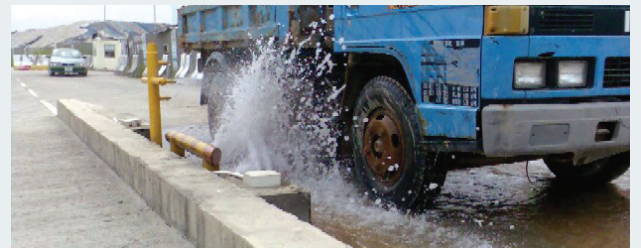
車輛離開工地前，須先清洗車輪 Wheel washing before leaving the site
