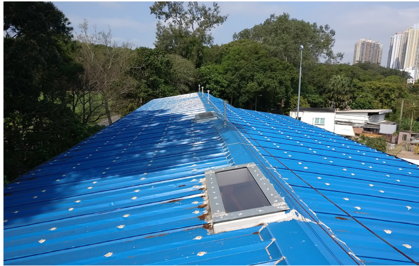
於地盤辦公室採用光井善用天然光 Installing Light Well at Roof of Site Office for Receiving Natural Light
