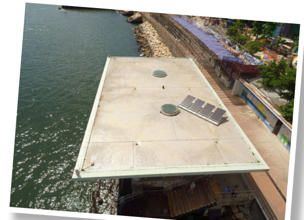
於荃灣公眾登岸台階的太陽能系統 Solar Energy System in Tsuen Wan Public Landing
