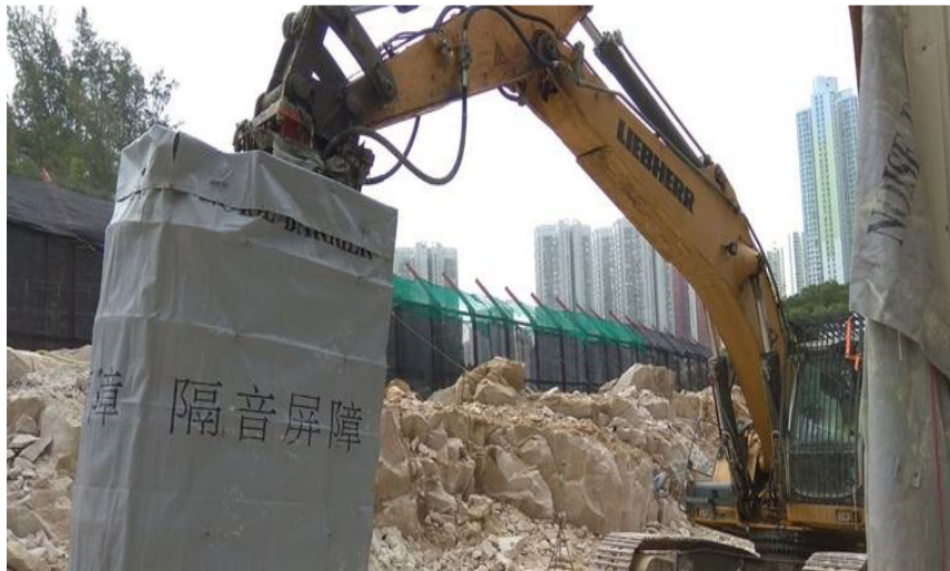
於打石工程採用度身定制的隔音屏障 Use of Tailor-Made Noise Barrier for Breaker
