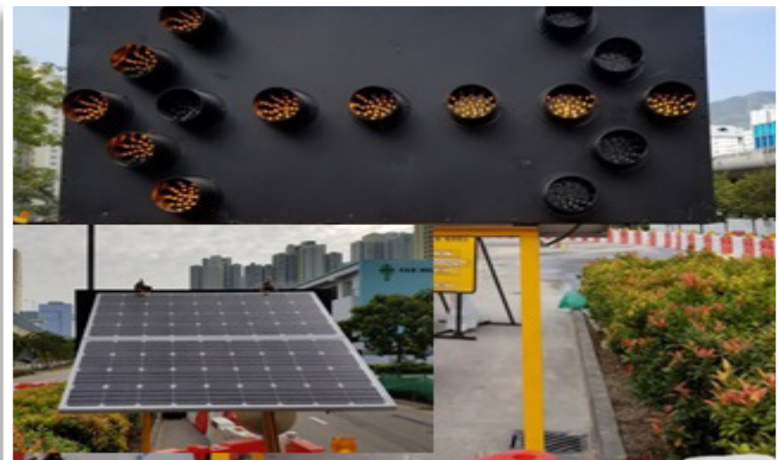
於臨時交通指示燈牌及警告燈安裝太陽電板作為照明電源及顯示 Installation of Solar Panels at Roof of the Site Accommodation and Temporary Traffic Signage/Warning Lanterns for Lighting and Display Purpose
