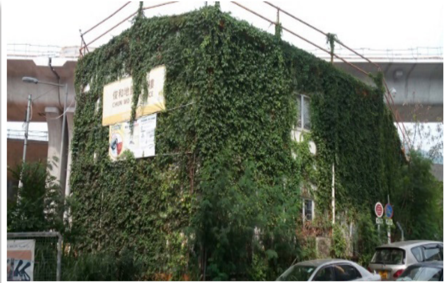
採用綠化外牆以減少工地辦公室的視覺影響和室內溫度 Adoption of Green Wall to Reduce the Visual Impact and Indoor Temperature of Site Office
