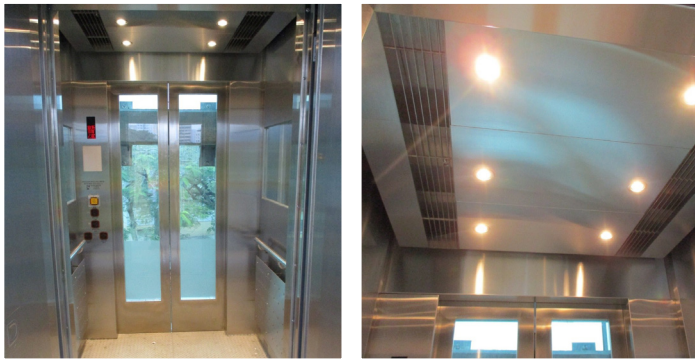
升降機內採用高效節能和耐用的LED照明系統 Adoption of Energy Efficient and Durable LED Lights in Lift Car
