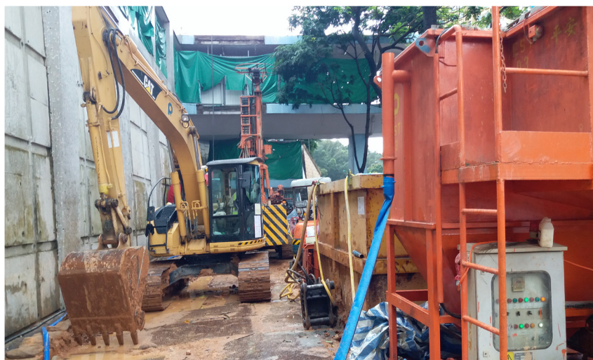
使用沉澱缸處理工地污水 Use of Sedimentation Tanks for On-Site Wastewater Treatment
