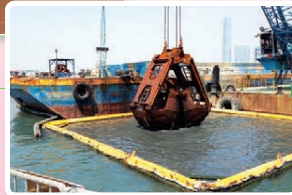
灣仔發展計劃第二期工程 Wan Chai Development Phase II 使用隔泥幕緩解疏浚工程對水質的影響 Use of silt curtain to mitigate impacts on water quality during dredging works
