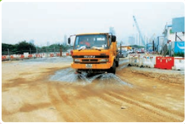
啟德發展計劃 Kai Tak Development 沿運料路灑水用以抑制泥塵 Watering along haul road for dust suppression
