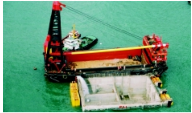
採用預製件方法建造海水泵房以減少建築廢料 Precasting Seawater Pumping Station to reduce Construction Waste
