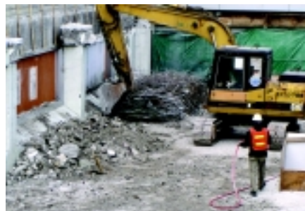
分揀物料以供循環再用 Separation of Materials for Recycling
