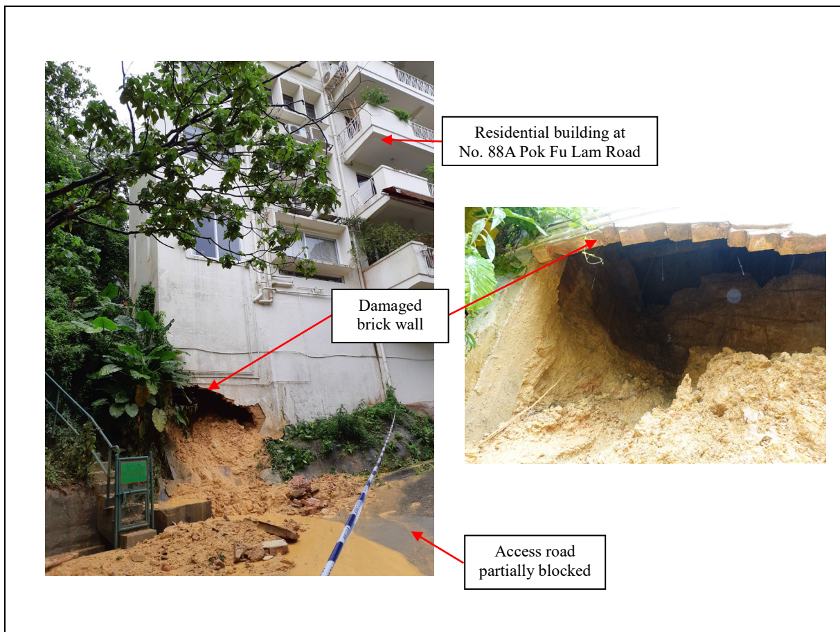
Figure 4.2 Views of the 26 August 2019 Landslide on a Cut Slope at No. 88A Pok Fu Lam Road, Hong Kong Island (Incident No. 2019/08/2488)
