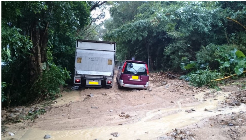
(a) A section of Fan Kam Road inundated by outwash debris
