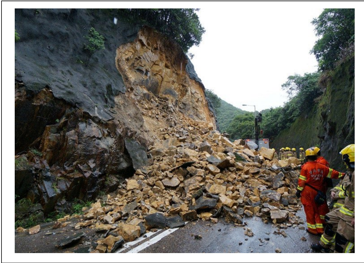
Figure 4.3 View of the 13 June 2017 Landslide on Slope No. 11SE-C/C148 at Tai Tam Road (Incident No. 2017/06/2028)
