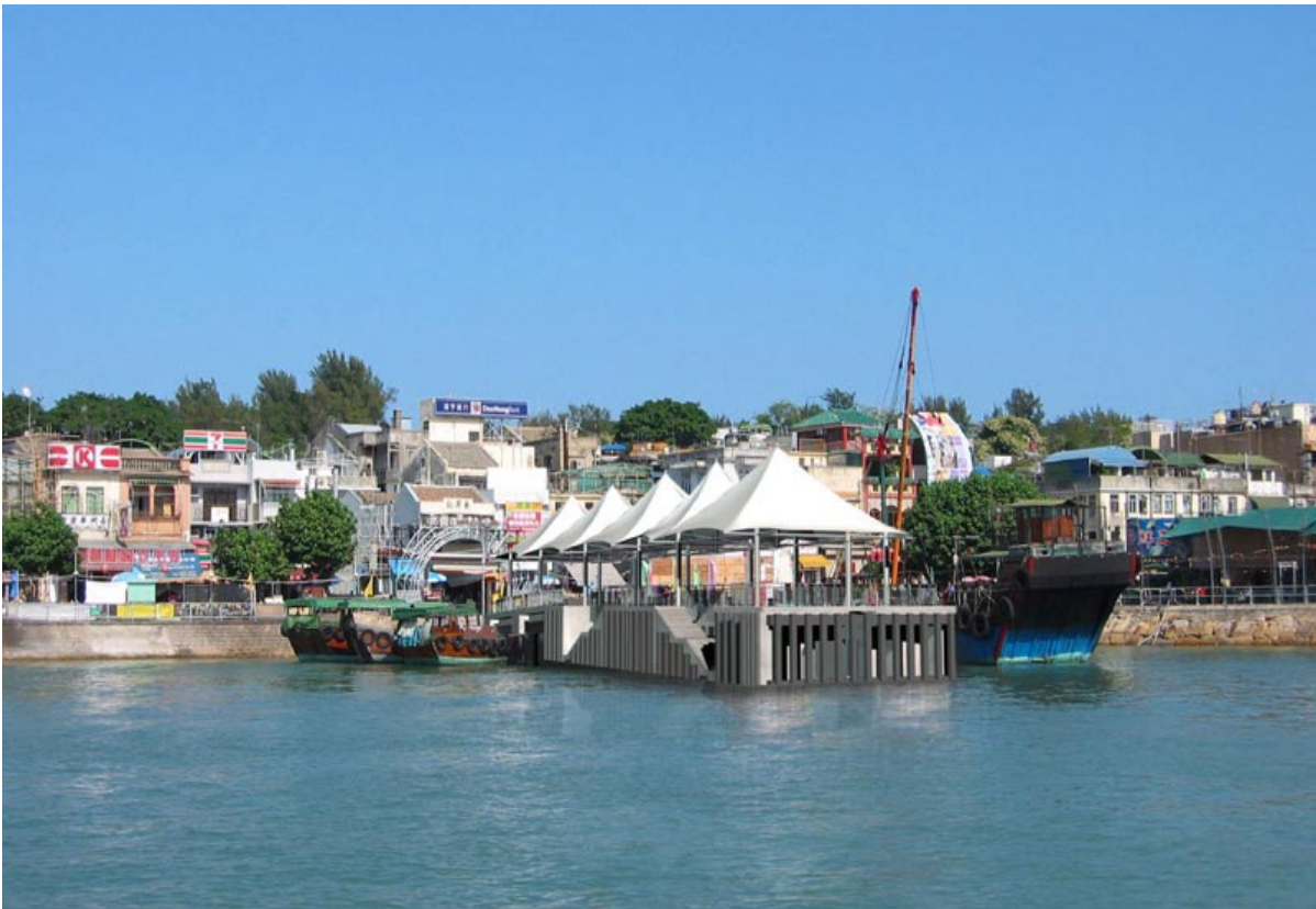
Plate 14 – Cheung Chau Public Pier
