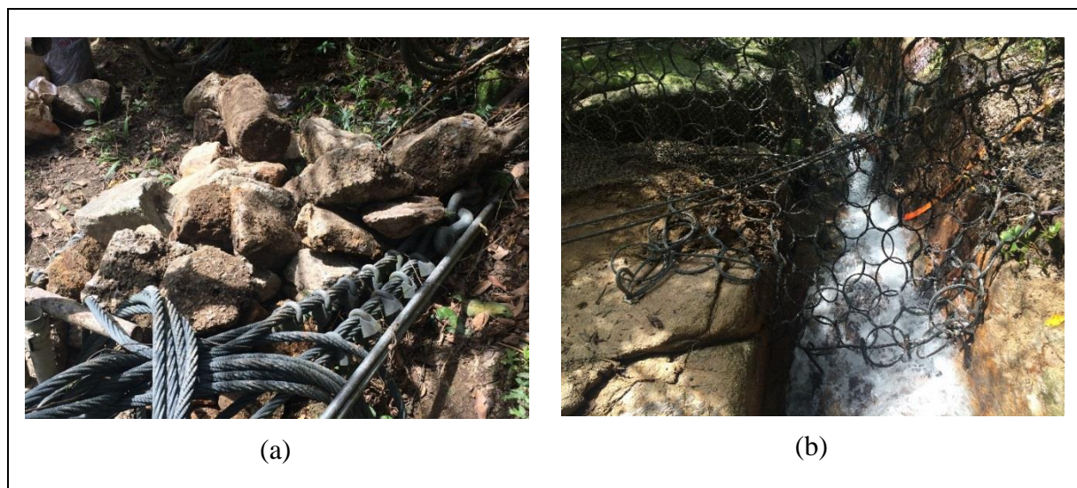
Figure A5 Photos Taken after Clearance of Trapped Stream Loads: (a) Boulders Removed from the Gully; and (b) Active Stream Flow Observed
