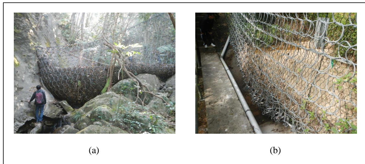
Figure 3.1 Other Cases of Trapping of Stream Loads by Flexible Barriers Traversing across Stream Course at: (a) Kwun Yam Shan; and (b) Fo Tan
