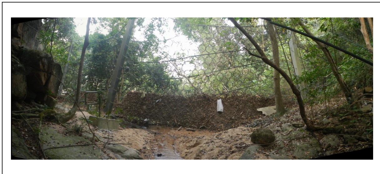
Figure 2.1 Overview of Flexible Barrier Trapped with Stream Loads at Shatin Hospital
