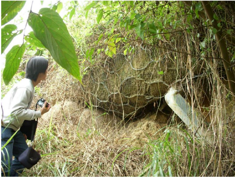
Figure 5.3 Capturing of Landslide Debris by a Flexible Barrier with Secondary Mesh in Jordan Valley (Kwan & Koo, 2015)
