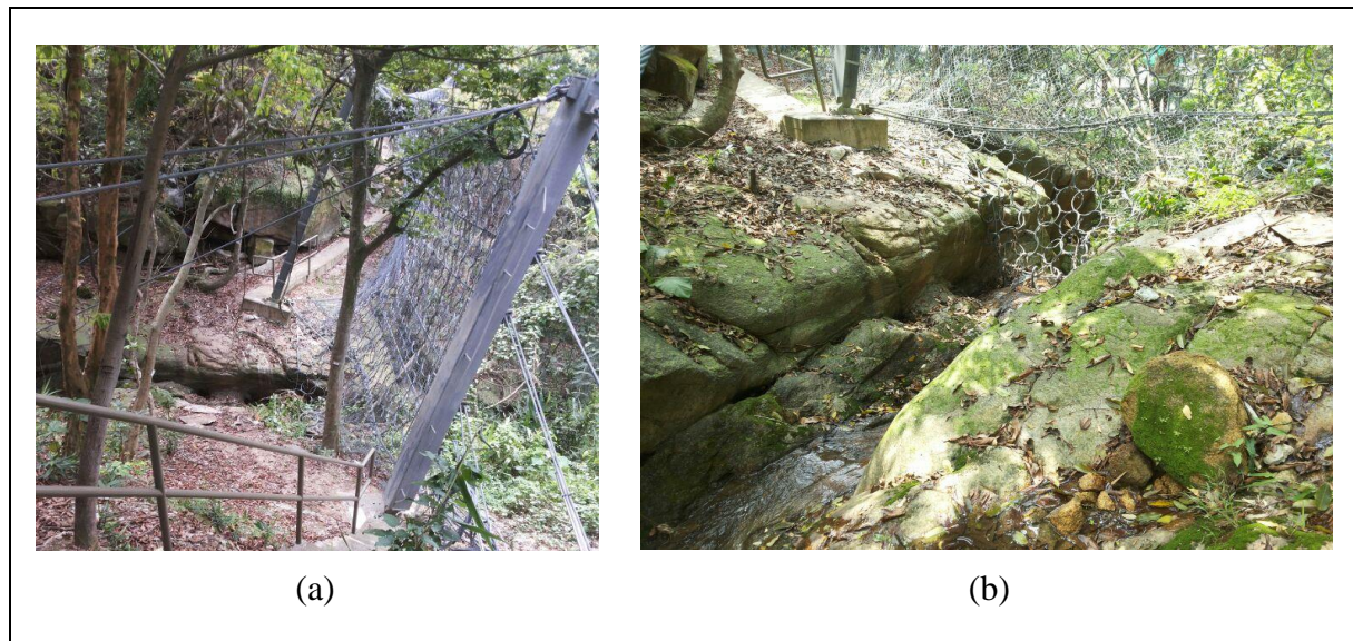
Figure A4 Photos of (a) the Flexible Barrier; and (b) Netting Details after Construction
