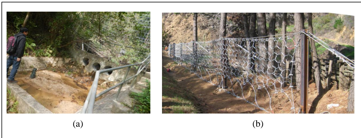
Figure 6.1 Examples of Detailing to Facilitate Passing of Stream Loads by Provision of: (a) Drainage; and (b) Enlarged Net Opening near the Bottom (Maccaferri, 2009)
