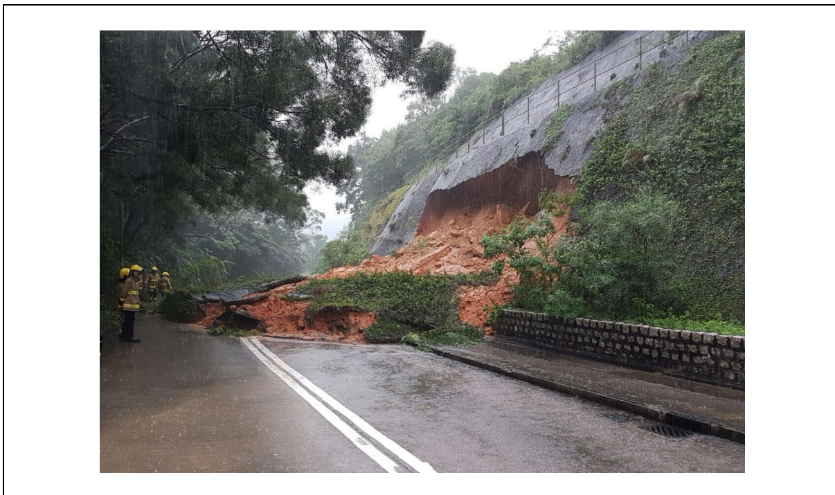
Figure 4.4 General View of the 7 September 2016 Landslide on Slope No. 13NE-A/C78 at South Lantau Road (Incident No. 2016/09/1917)
