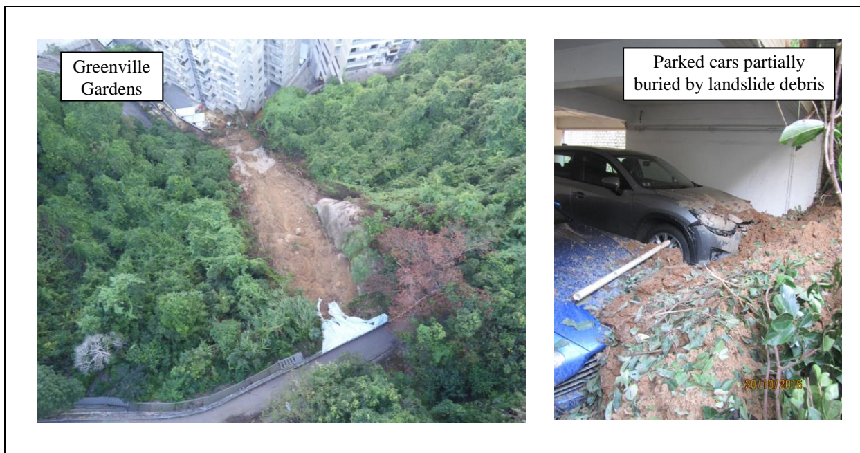
Figure 4.2 Views of the 19 October 2016 Landslide on the Natural Hillside behind Greenville Gardens (Incident No. 2016/10/1941)
