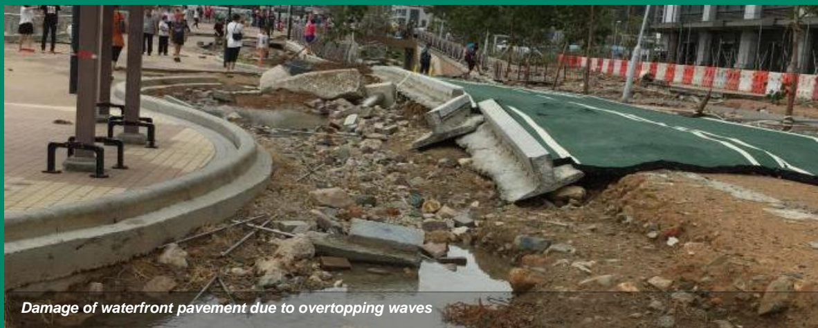
Coastal flooding due to spreading of water from overtopping waves
