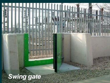
Demountable flood barrier at open area
