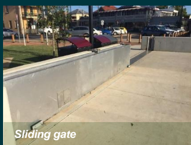
Demountable flood barrier at ground opening
