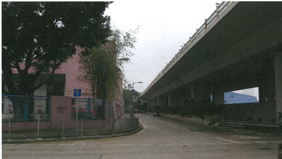
Figure 5.4: Existing Columns Supporting the Kai Fuk Road Flyover
