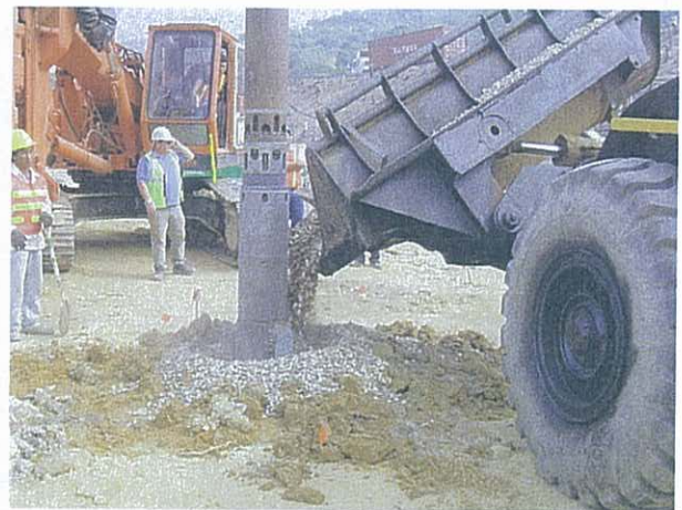
Top Feed Installation
