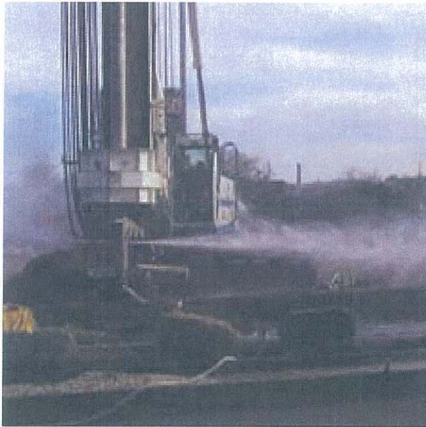
Photos of Formation of Lime Columns
