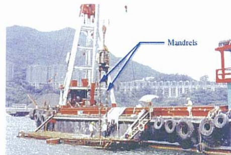
Installation of Drains on a Barge
