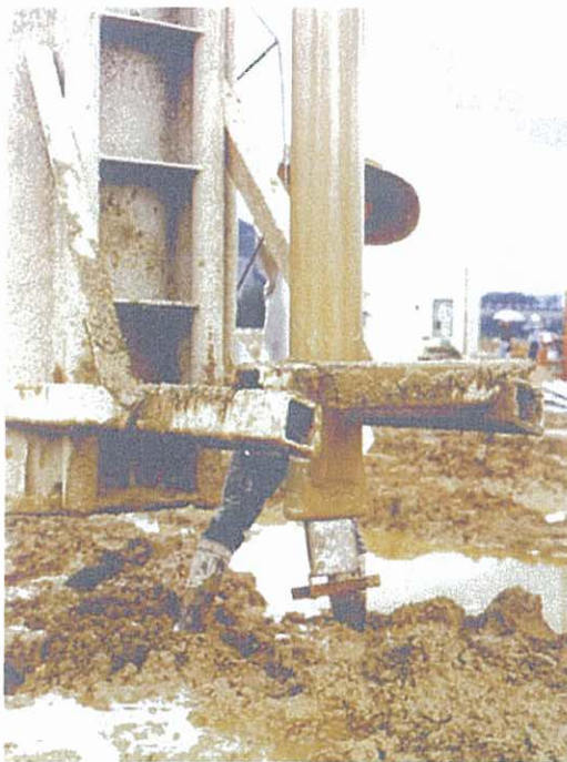
The drain which is placed inside the mandrel with tip anchor.
