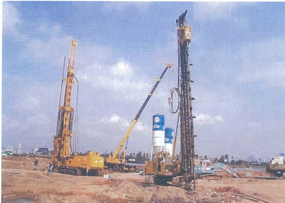
Photos of Deep Cement Mixing (Land-based)
