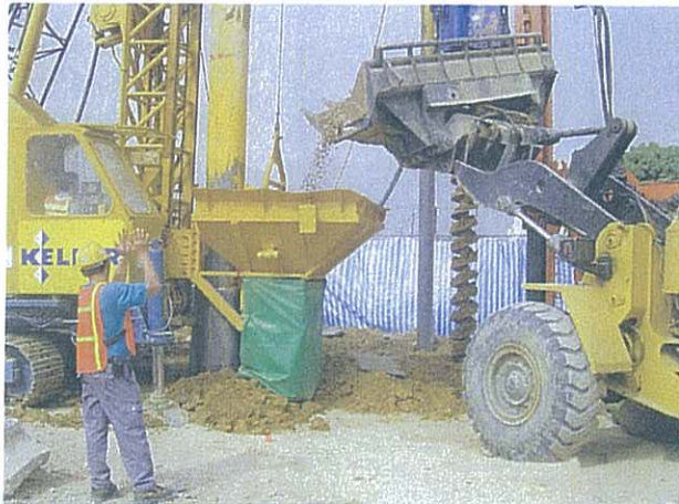
Bottom Feed Installation
