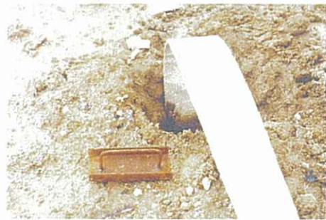
The details of band drain and tip anchor.
