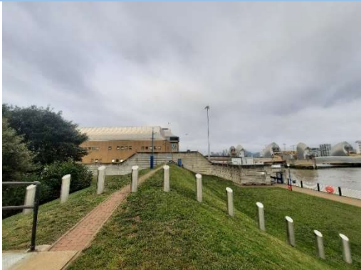
Addition of berm behind shoreline to raise height of shoreline in future in place of raising whole formation level.
