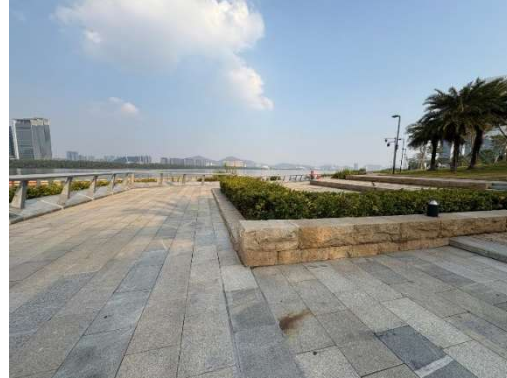
Stepped or sloped surface to enable runoff and maintain access at different levels.
