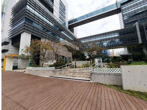
High formation level to mitigate sea water inundation.
