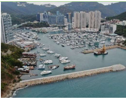
Future – PAA may consist of raised wave wall height or large scale coastal structure, such as breakwater.
