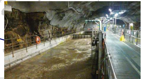
Stanley Sewage Treatment Works (1995)
