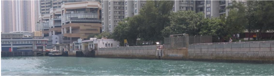
Vertical concrete seawall at Sai Wan Ho Pier
