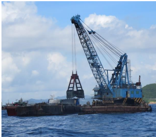
Dredging marine deposits
