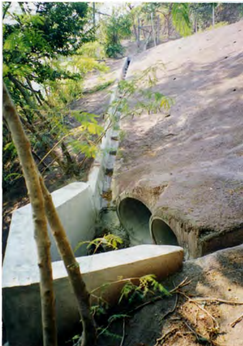
(c) Cross Road Drain and Hard Wearing and Impermeable Slope Surface on the Downhill Side of a Road
