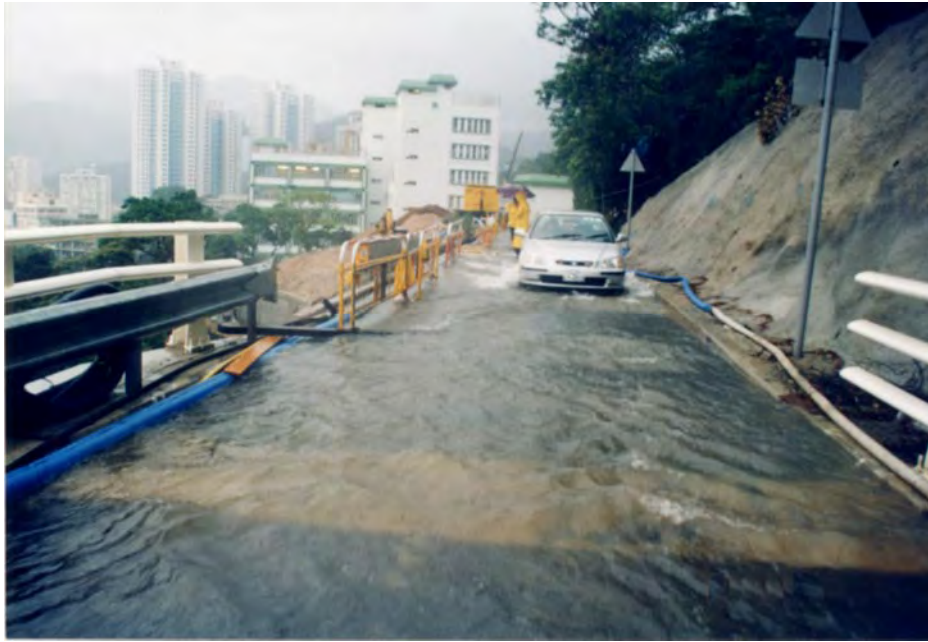
Plate 5.1 Surface Runoff Channelising along a Road
