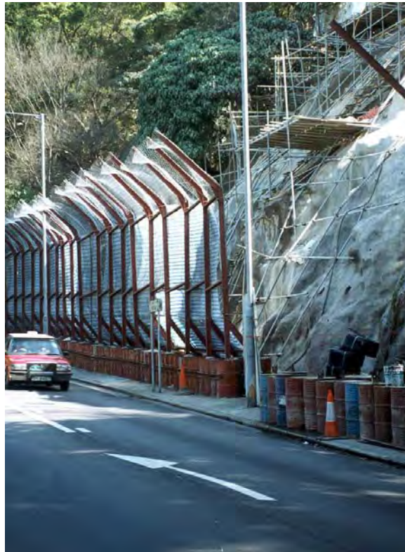
Plate 7.1 Typical Temporary Protective Fences in Hong Kong
