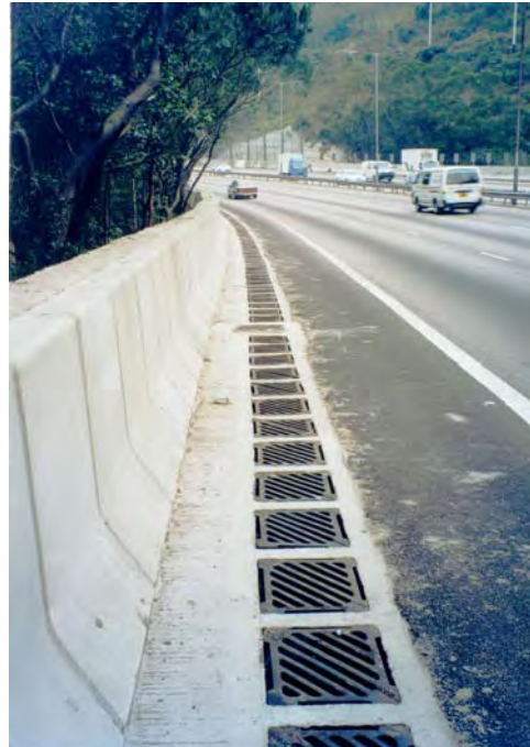
(d) Roadside Channel with Grating Covers to Intercept Road Surface Runoff
