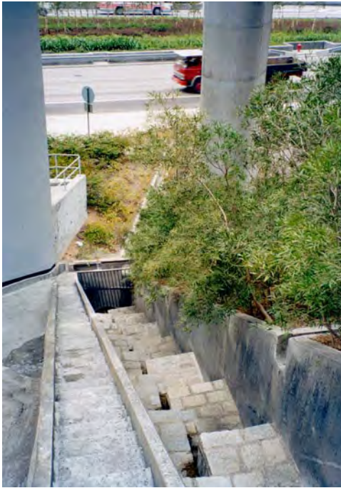
(a) Trash Grill at Inlet of Cross Road Drain to Minimise Chance of Blockage
