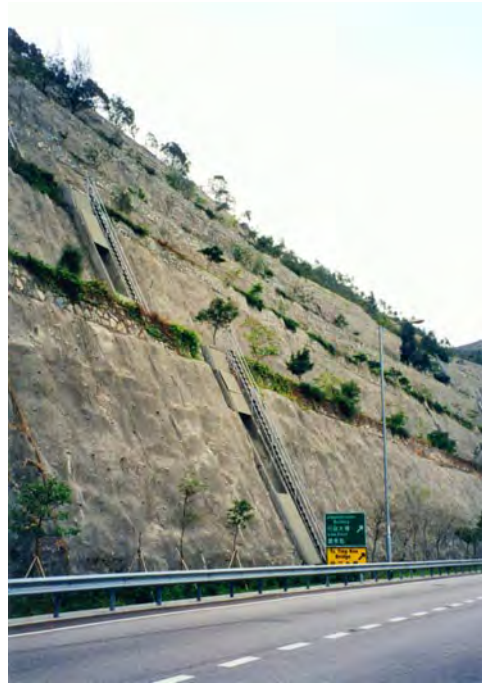
(b) Cascade with Cover to Carry Water Down a Steep Rock Slope
