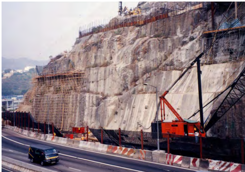
Plate 7.2 Specialised Rockfall Fence
