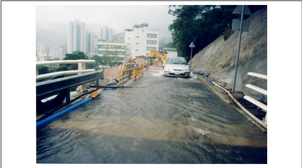
Plate 5.1 Surface Runoff Channelising along a Road
