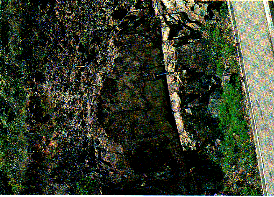
Plate 1.8 - Cut Slope through Weathered Volcanic Rock Showing Zone B Overlying Zone D : Zones A and C are Absent
