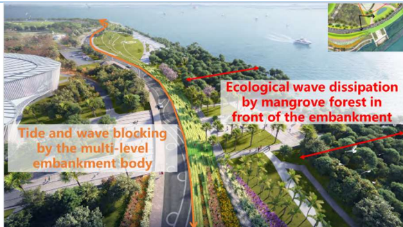
NbS may be designed to dissipate wave energy.
