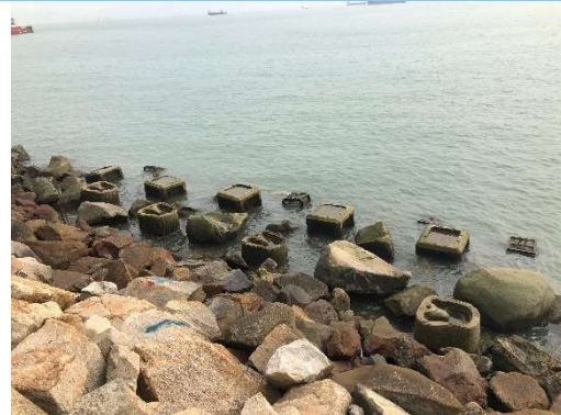
Large precast habitat-enhancement units can also be deployed in sub-tidal or inter-tidal areas, helping dissipate wave energy as well as supporting a variety of marine species. Pools can be an effective way of providing habitats for intertidal organisms in artificial environments.
