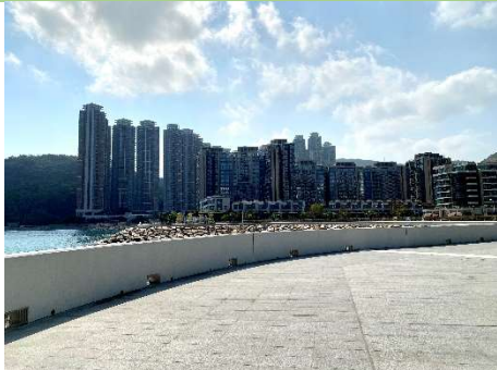
Wave wall to minimise overtopping wave.
