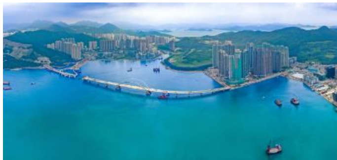
Tseung Kwan O – Lam Tin Tunnel and Cross Bay Link
