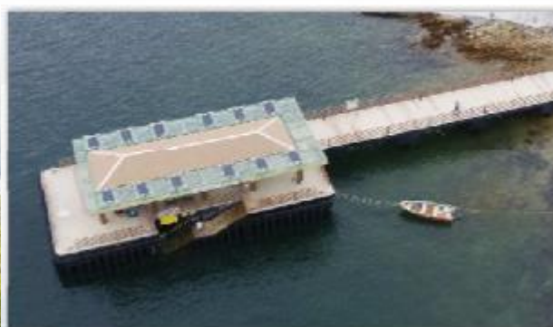
Reconstruction of Sharp Island Pier
