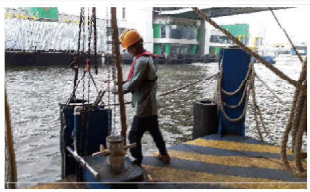
Fender repair works at the pier
