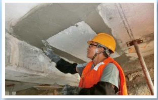
Patch repair at suspended deck of pier
