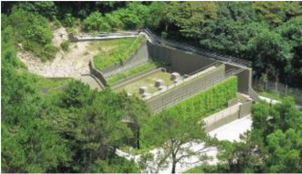
Greening measures on concrete rigid barrier at North Lantau Highway
