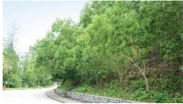
Slope upgrading works with greening measures at South Lantau Road
