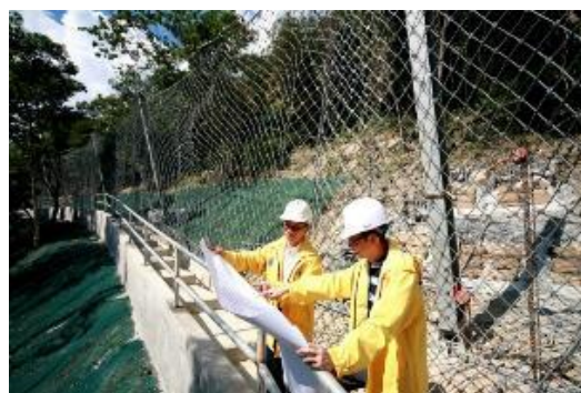
Investigation works under LPMitP
