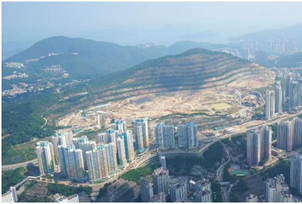
A view of the rehabilitated Anderson Road Quarry
