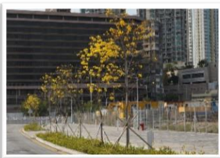
Kai Tak Development Infrastructure Works at Former North Apron Area
