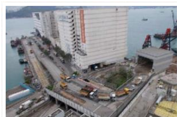
Chai Wan Public Fill Barging Point
