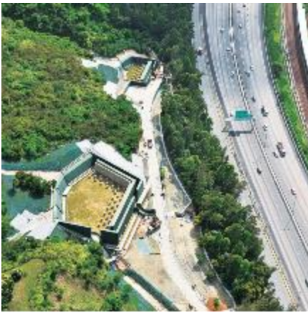
Check dams protecting North Lantau Highway
