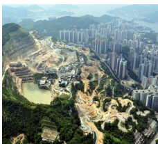
Control of site formation works
