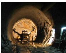
Rock cavern & underground space development
