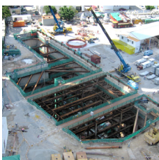
Control of deep excavations
