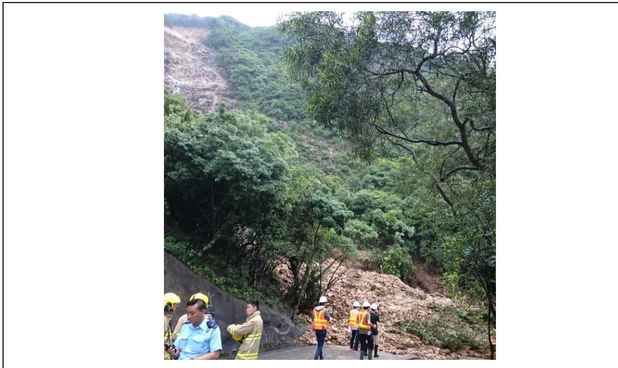
Figure 1.3 View of the Debris Deposited on Sai Kung Sai Wan Road Resulting in Complete Road Blockage (Photograph taken on 21 May 2016 by GEO Emergency Duty Officer)
