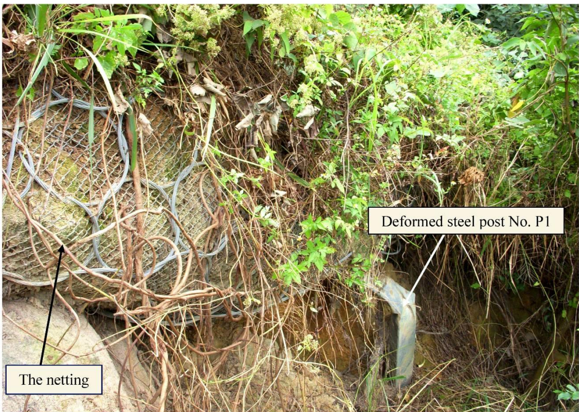
Plate 5 – Steel Post No. P1 was Pushed Forward Together with the Netting
