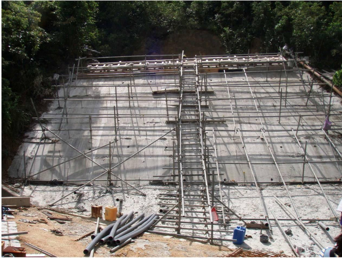
Plate 12 – Remedial Works for the Landslide Scar
