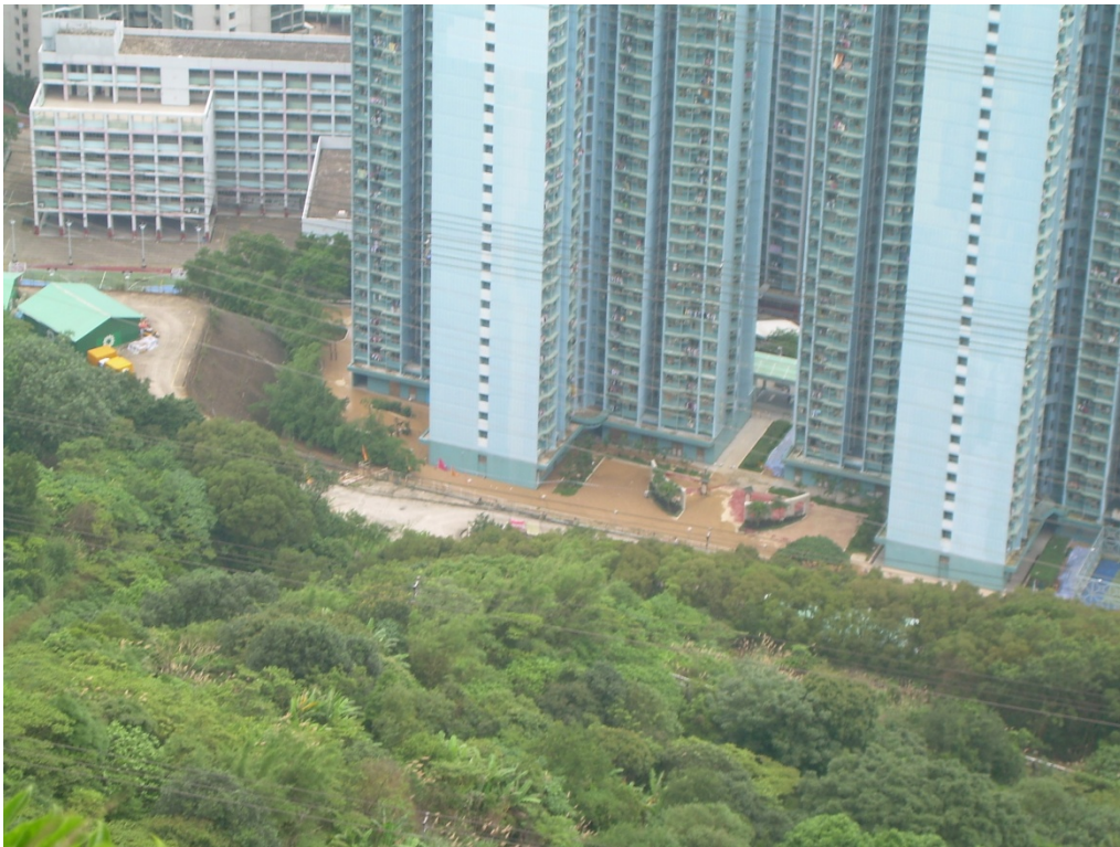
Plate 6 - General View of Outwash Debris within Tsz Ching Estate (Photograph taken on 9 June 2008)
