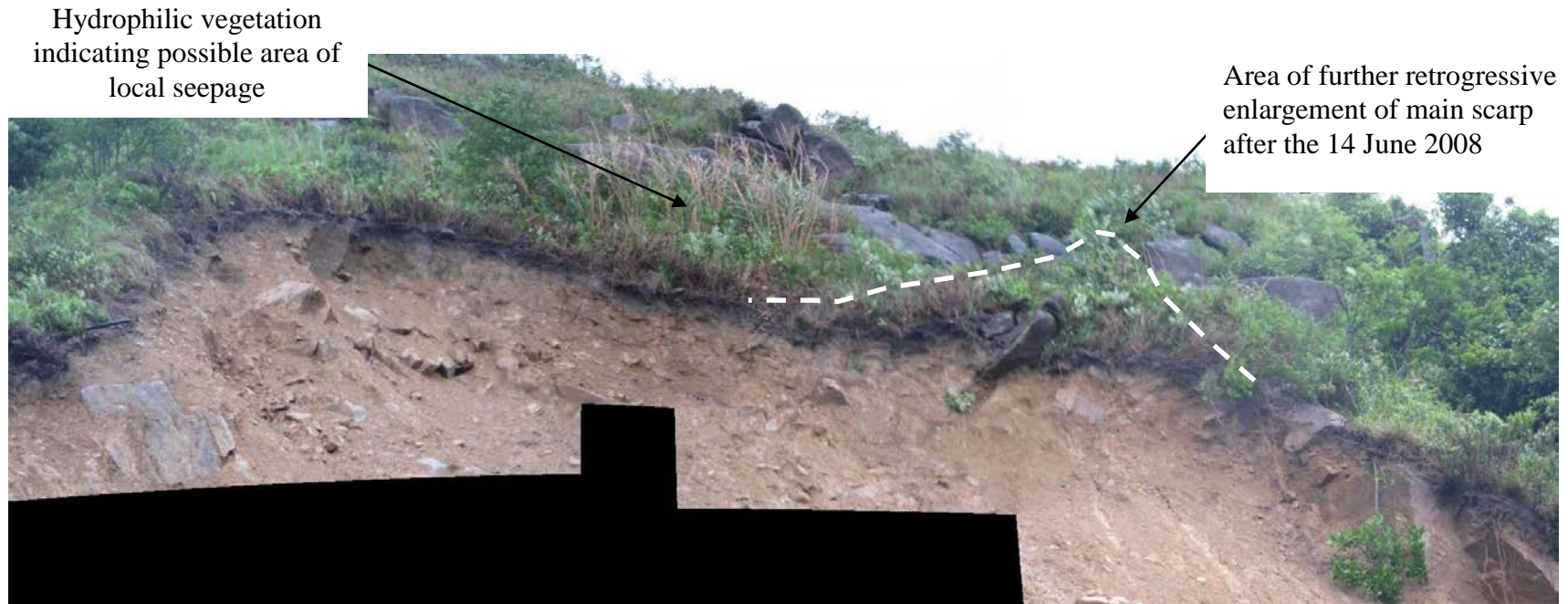
Plate 23 - Detailed Panoramic View along the Crown of the 7 June 2008 Landslide (Photograph taken on 13 June 2008)
