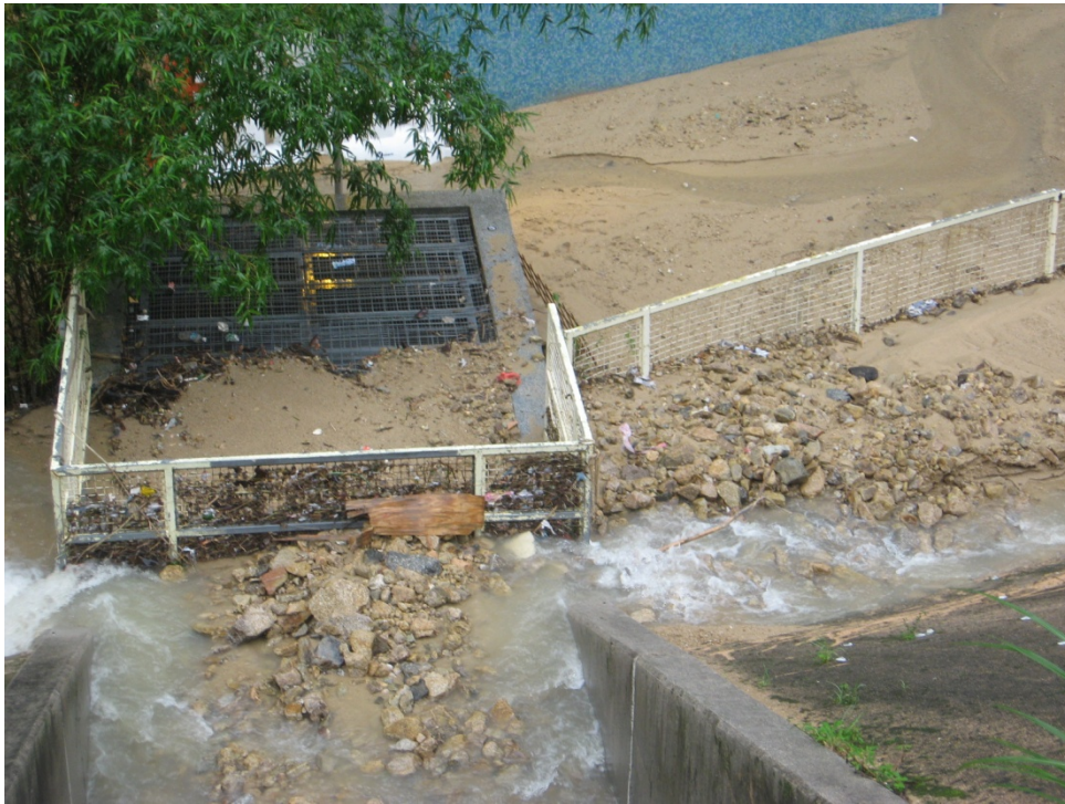
Plate 12 - Debris Outwash Accumulated behind Fence above Tsz Ching Estate after the 12 July 2008 Rainstorm (Photograph taken on 12 July 2008)
