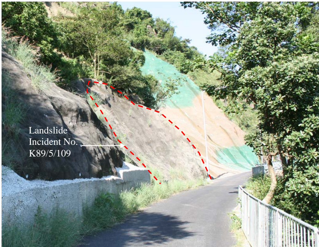
Plate 20 - Recent Photograph Showing the Shotcrete Covered Scar from Landslide Incident No. K89/5/109 (Photograph taken on 24 August 2009)
