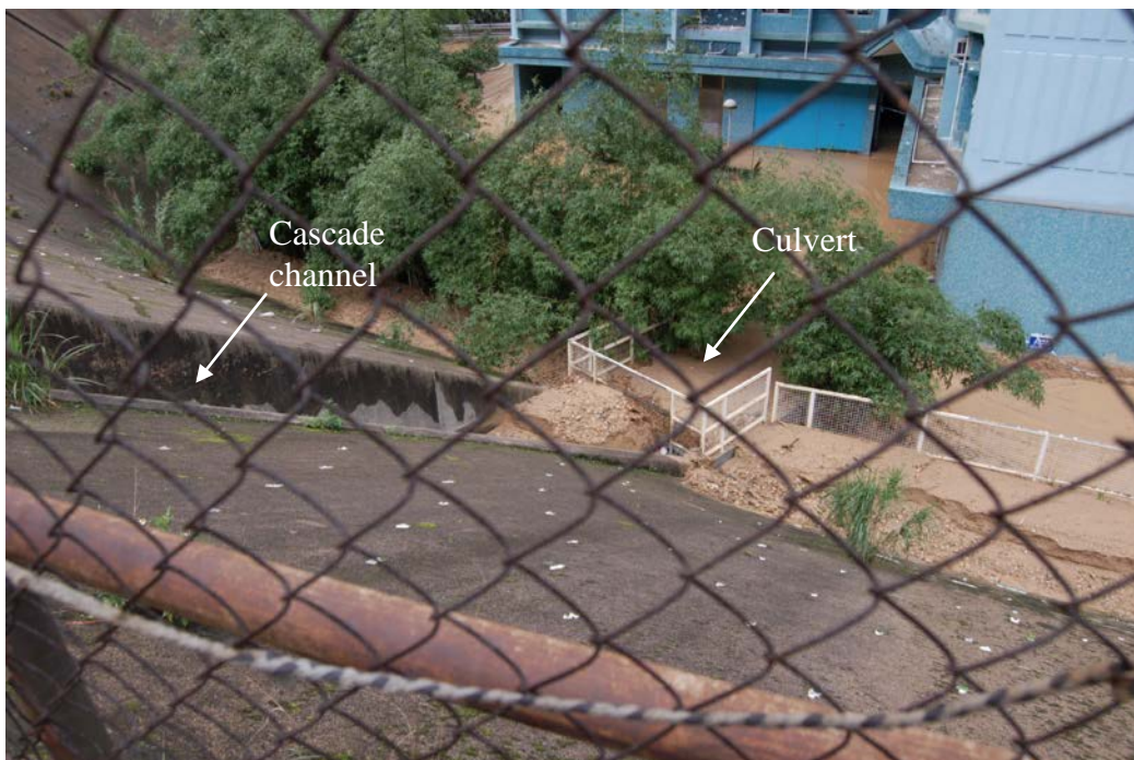
Plate 7 - Debris Outwash Accumulated behind Fence above Tsz Ching Estate (Photograph taken on 10 June 2008)
