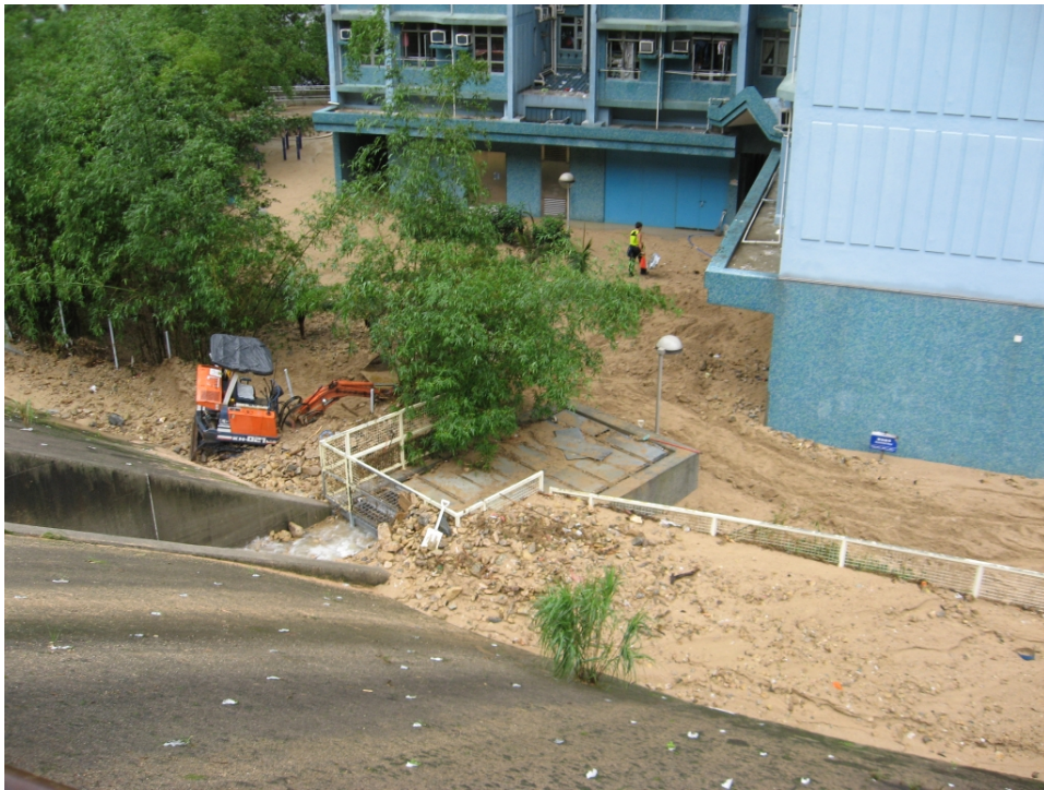
Plate 10 - Debris Outwash Accumulated behind Fence above Tsz Ching Estate after the 13 and 14 June 2008 Rainstorm (Photograph taken on 16 June 2008)
