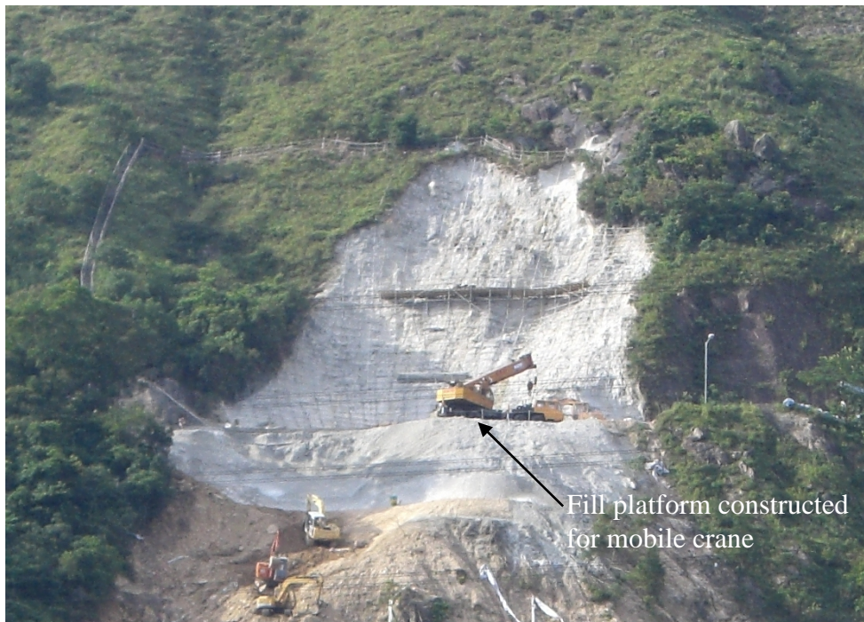
Plate 13 - Ongoing Remediation Work of the Source Area (Photograph taken on 22 July 2008)
