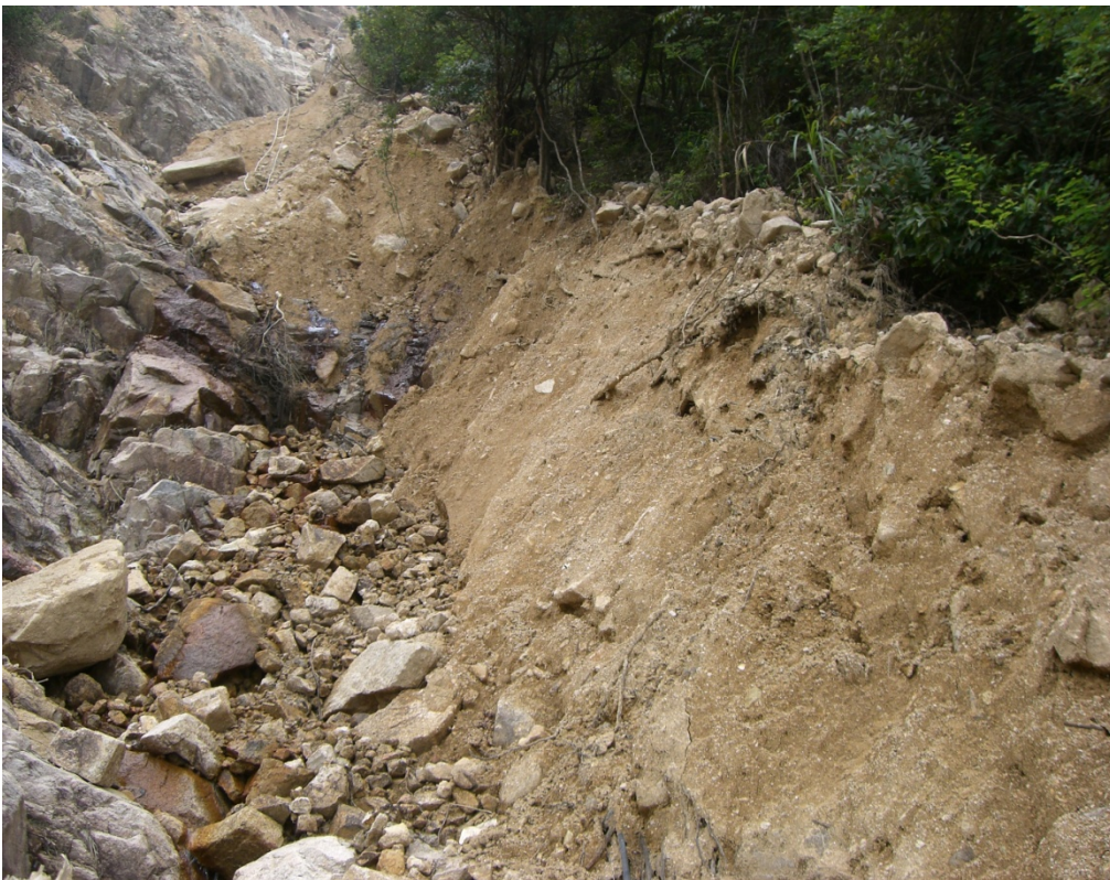
Plate 33 - Debris within Channelised Debris Flow Path at about CH170 (Photograph taken on 29 July 2008)
