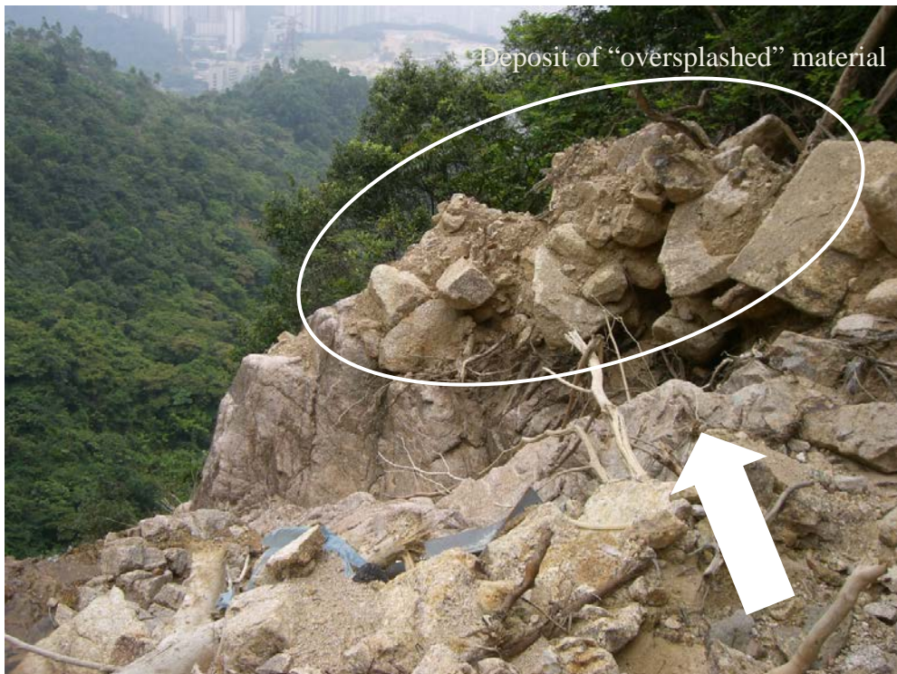
Plate 36 - Deposit of "Oversplashed" Debris at about CH170 (Photograph taken on 29 July 2008)
