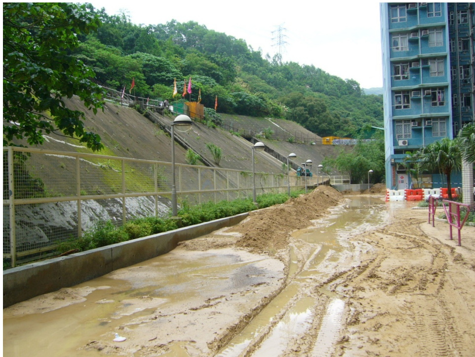
Plate 9 - Debris Outwash within Tsz Ching Estate after the 13 and 14 June 2008 Rainstorm (Photograph taken on 15 June 2008)
