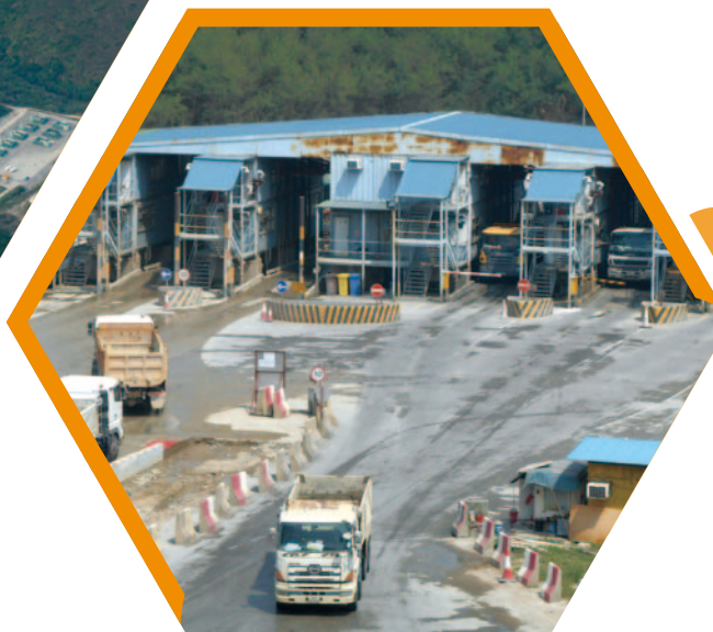
將軍澳第137區公眾填料接收設施 – 磅橋 TKO Area 137 Public Fill Reception Facility – weighbridges
