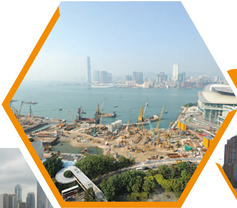
香港會議展覽中心西面正全速進行土地平整工程 Land formation works at the west of Hong Kong Convention and Exhibition Centre in full swing
