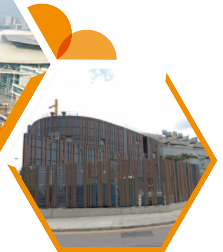
重置的海水抽水站 Reprovisioned salt water pumping station
