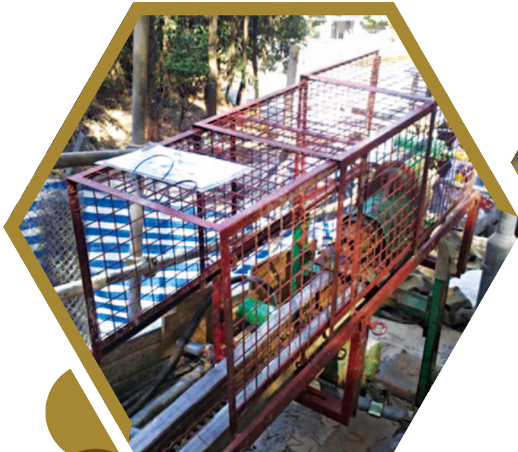
為鑽孔機提供護罩 Provision of protection guard for drilling machine
