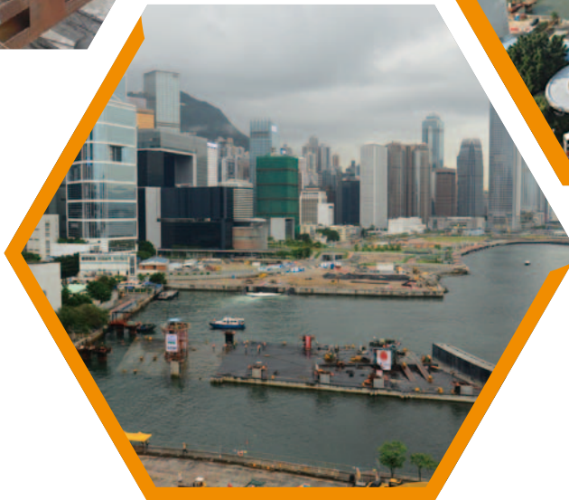
港鐵荃灣線過海隧道上方安裝巨型預製結構 Installation of gigantic precast structure above the MTR Tsuen Wan Line tunnel
