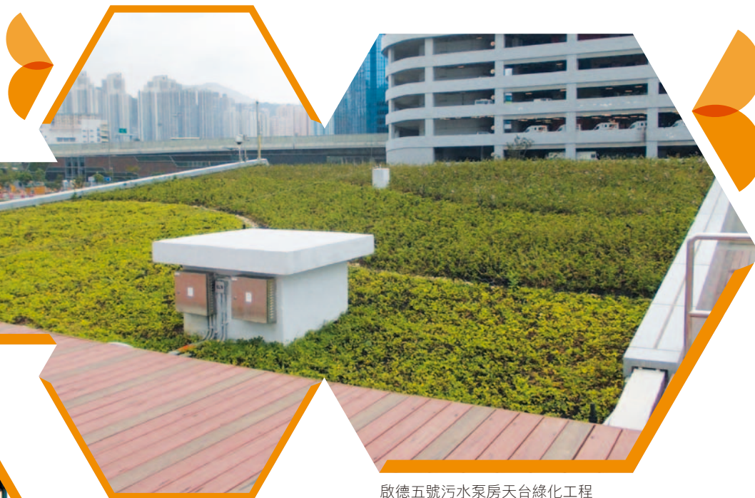
啟德五號污水泵站天台綠化工程 Roof greening works at Kai Tak No. 5 Sewage Pumping Station
