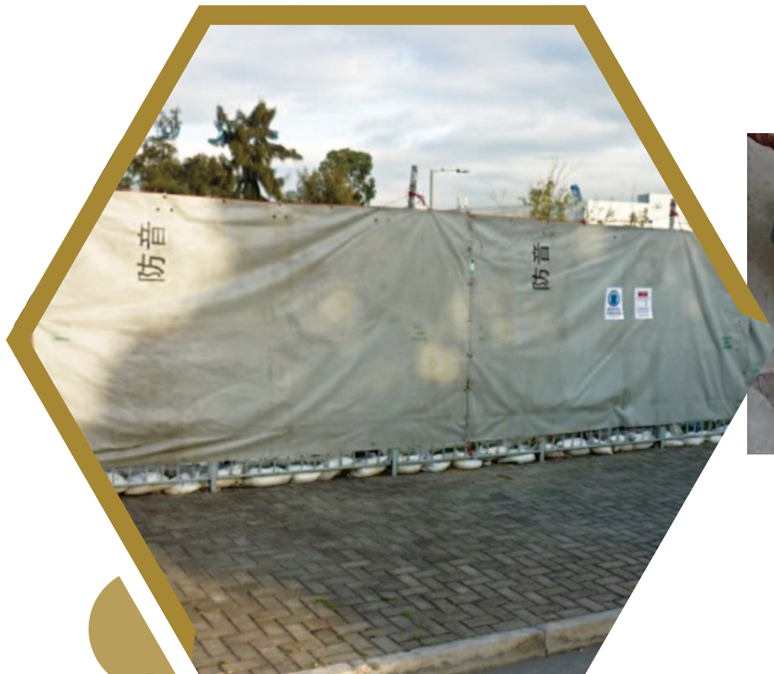
採用臨時隔音屏障以減低噪音 Provision of temporary noise barrier to reduce noise emission
