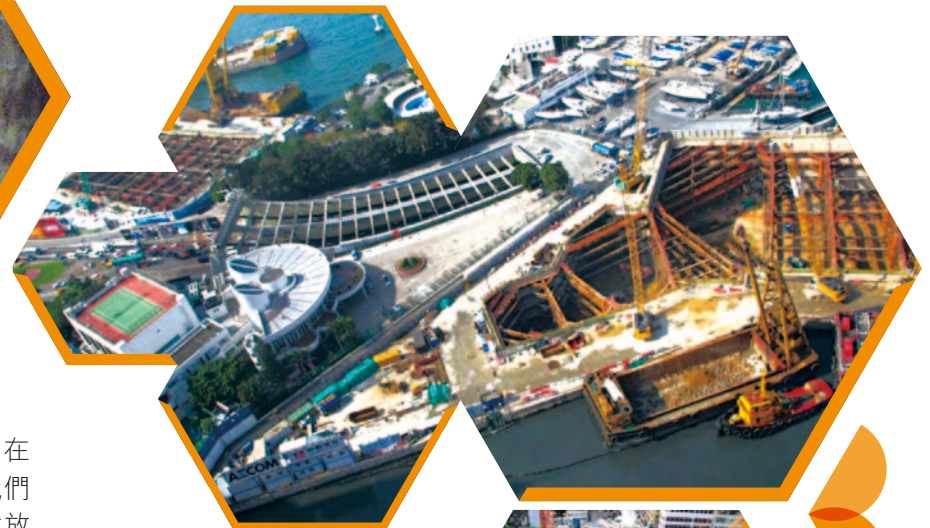
中環灣仔繞道 – 於現有的海底隧道底下順序開挖 Central-Wan Chai Bypass – Sequential excavation underneath Cross Harbour Tunnel
