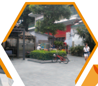
大澳—涌河堤建造工程已完成 Construction of riverwall at Yat Chung of Tai O was completed
