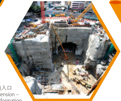
中環灣仔繞道 – 於現有的海底隧道底下順序開挖 Central-Wan Chai Bypass – Sequential excavation underneath Cross Harbour Tunnel
