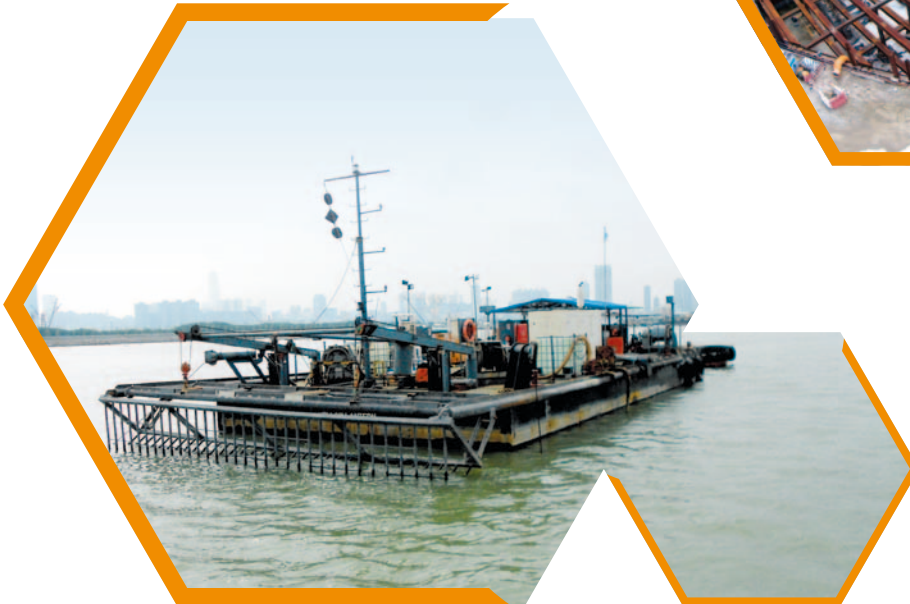
啟德明渠進口道與觀塘避風塘的生物除污工程 Bioremediation treatment at Kai Tak Approach Channel and Kwun Tong Typhoon Shelter
