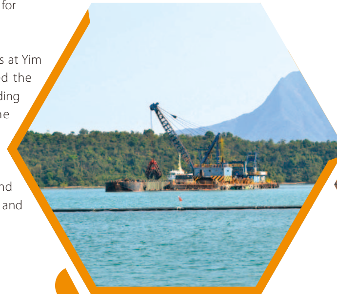
鹽田仔(東)養魚區的清除海床沉積物工程 Sediment removal works at Yim Tin Tsai (East) Fish Culture Zone
