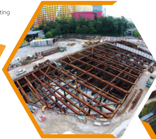
進行中的啟德明渠重建及改善工程，完成後將能抵禦重現期為200年一遇的水浸 Reconstruction and upgrading of Kai Tak Nullah in progress, which can withstand flooding with a return period of 1 in 200 years upon completion
