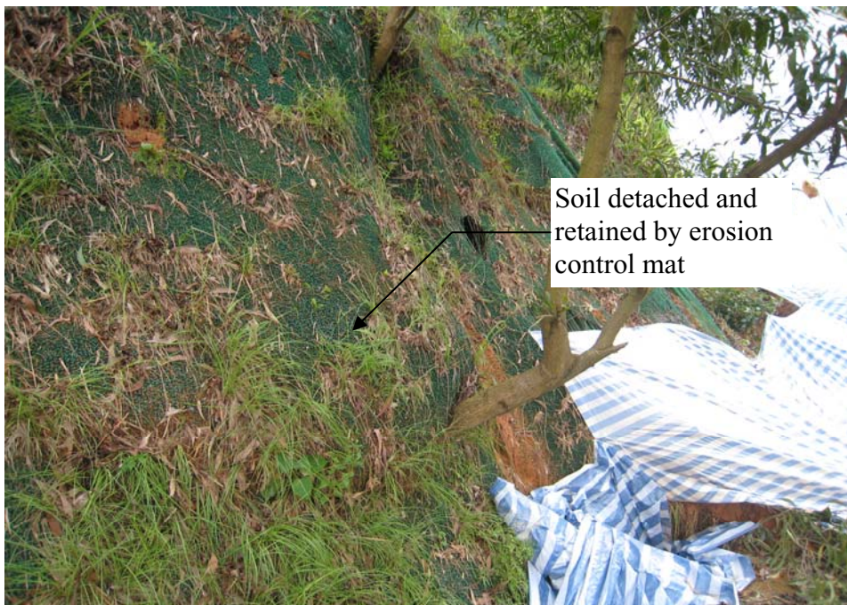
Figure 5.3 View of the Minor Detachment on the West (Photograph taken on 19 June 2008)
