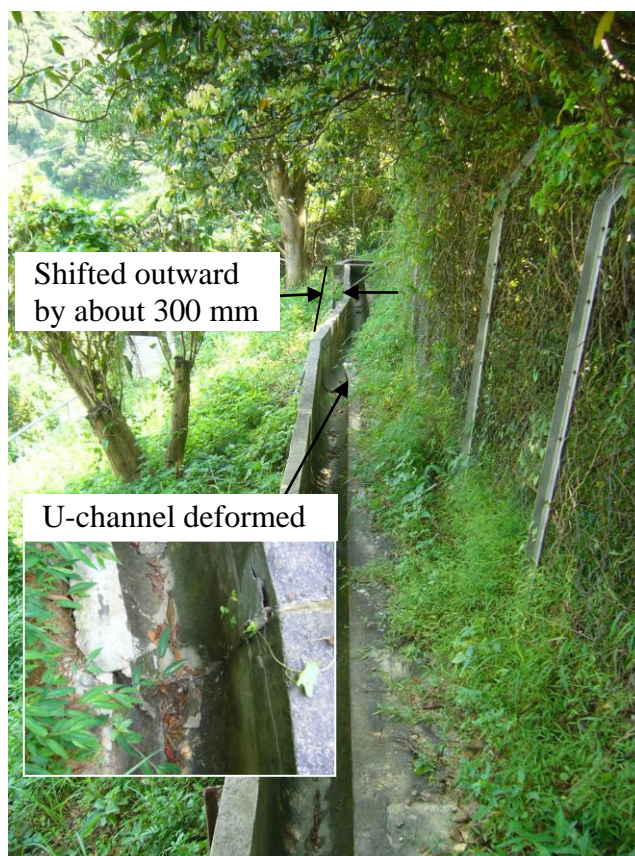
Plate 8 - Deformed Upper 300 mm U-channel near the Eastern End of Slope No. 6NE-B/C44 Looking East (Photograph taken on 26 September 2006)
