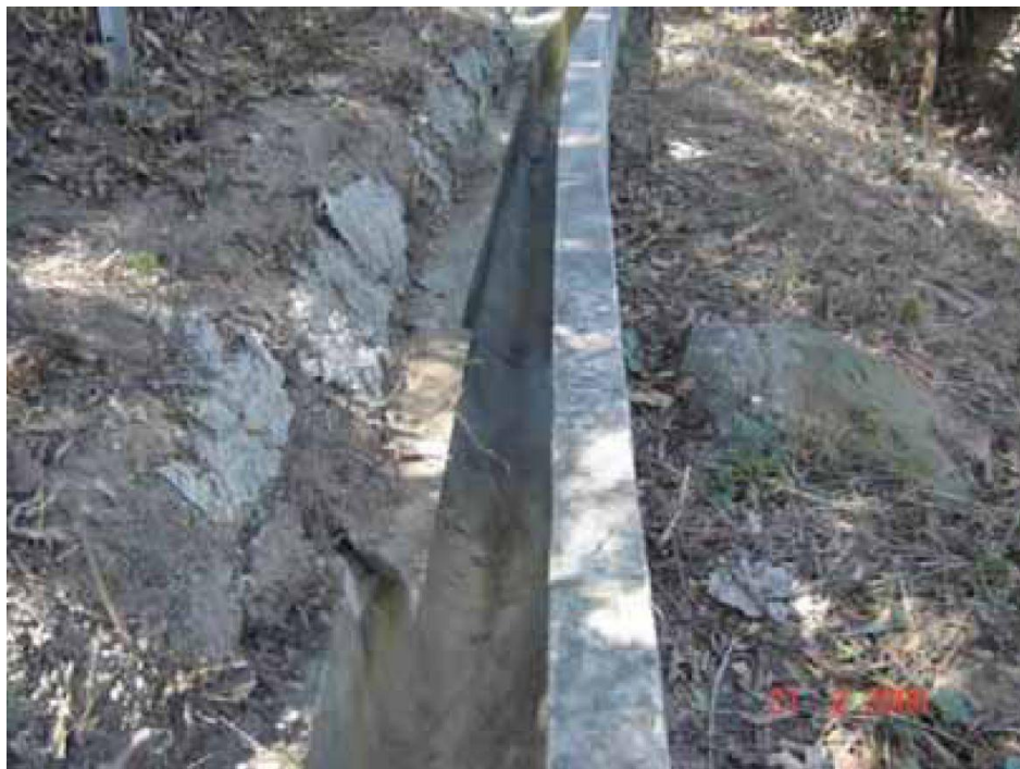
Plate 4 - Cracked Upper 300 mm U-channel of Slope No. 6NE-B/C44 (Photograph taken by OAP on 21 February 2006)
