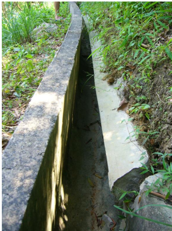
Plate 12 - Deformed Upper 300 mm U-channel (Photograph taken on 26 September 2006)
