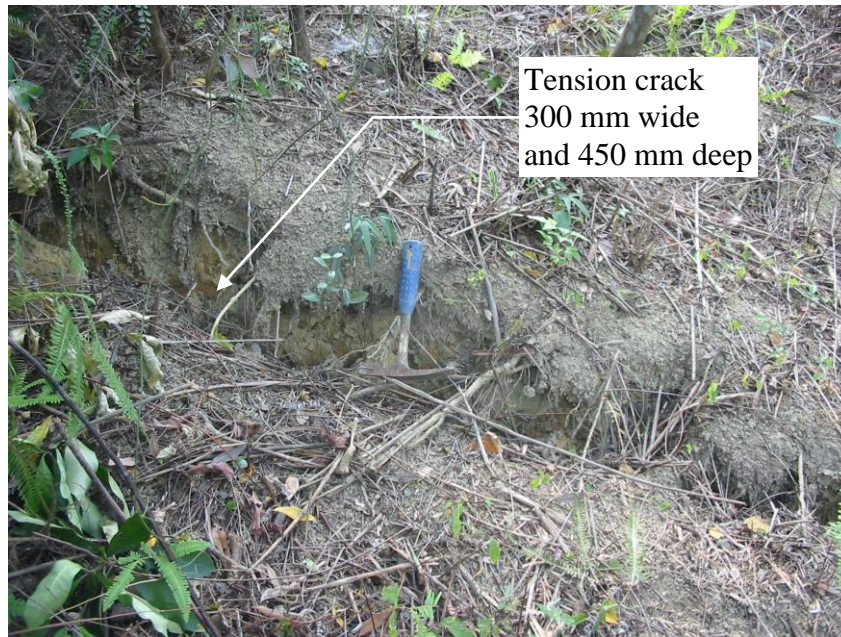
Plate 13 - Tension Crack on Area above Slope No. 6NE-B/C44 (Photograph taken on 19 November 2007)
