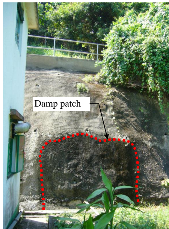
Plate 14 - Damp Patch on Shotcrete Surface (Photograph taken on 26 September 2006)
