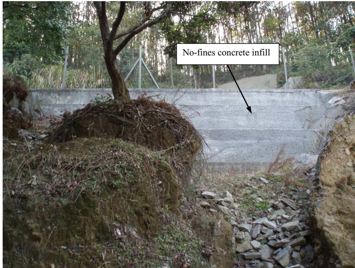
Plate 13 - General View of Remedial Works to Scar 3 on Slope No. 6SE-B/F69 (Photograph taken on 28 November 2007 by HCL)
