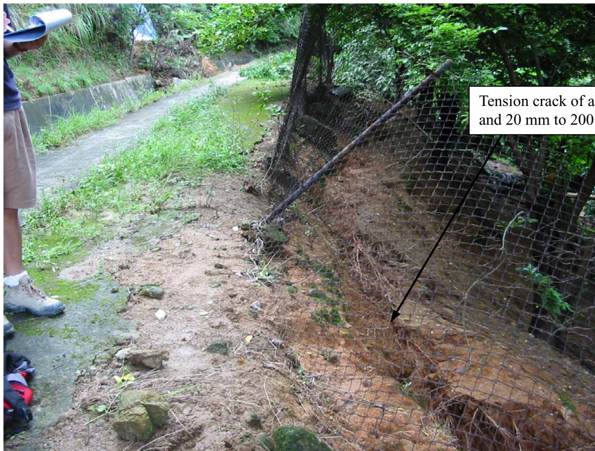
Plate 5 - Tension Crack at Crest of Slope No. 6SE-B/F69 (Photograph taken on 21 August 2005 by MGSL)
