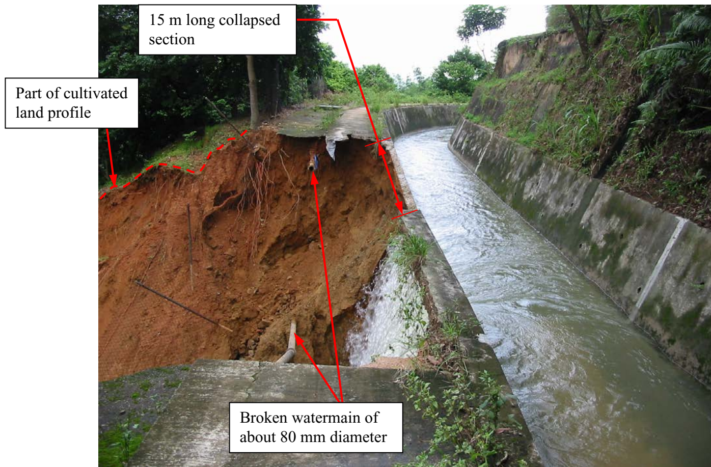
Plate 8 - Water Cascading Over Collapsed Section of Catchwater (Photograph taken on 21 August 2005 by MGSL)
