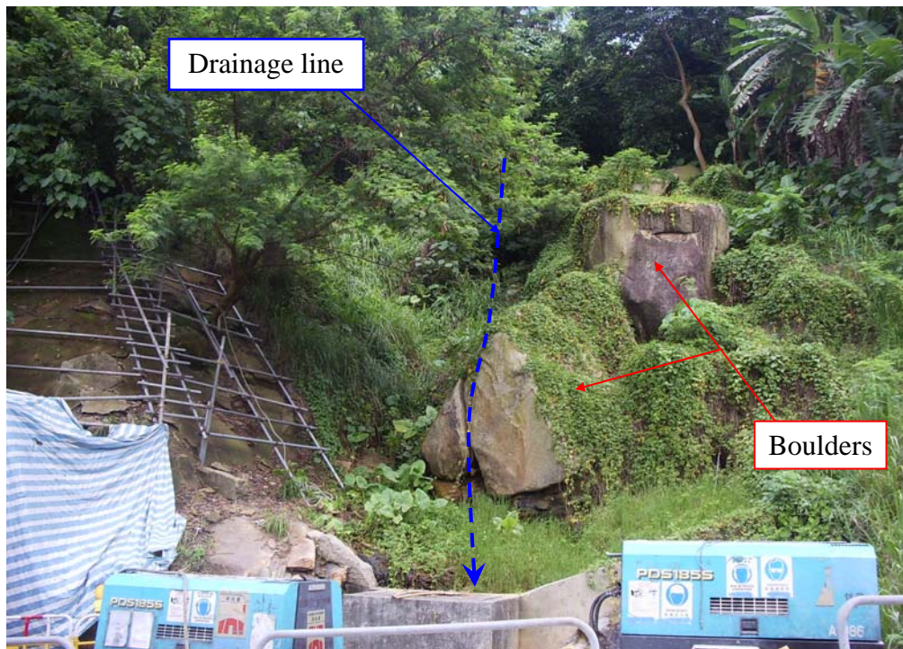
Plate 6 - Intercepted Drainage Line with Large Boulders (Photograph taken on 10 June 2008)
