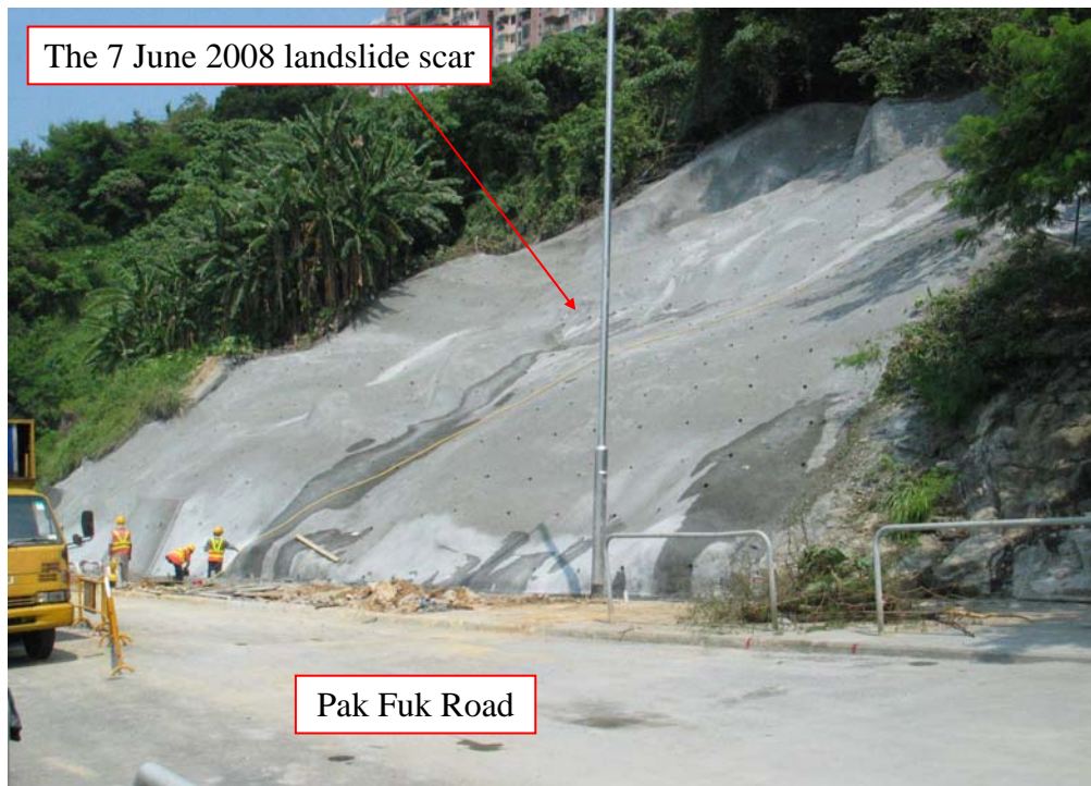
Plate 8 - The 2008 Landslide Scar after Completion of Emergency Repair Works (Photograph taken on 23 June 2008)
