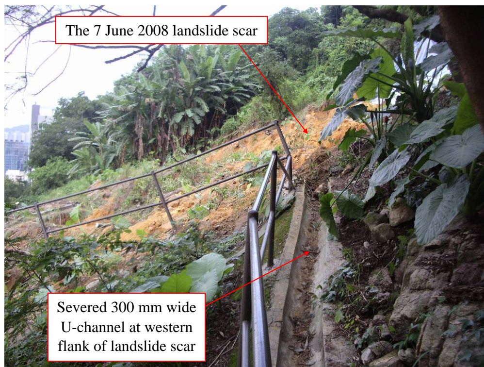
Plate 19 - Severed Drainage Channel at Mid-height of the Slope (Photograph taken on 10 June 2008)
