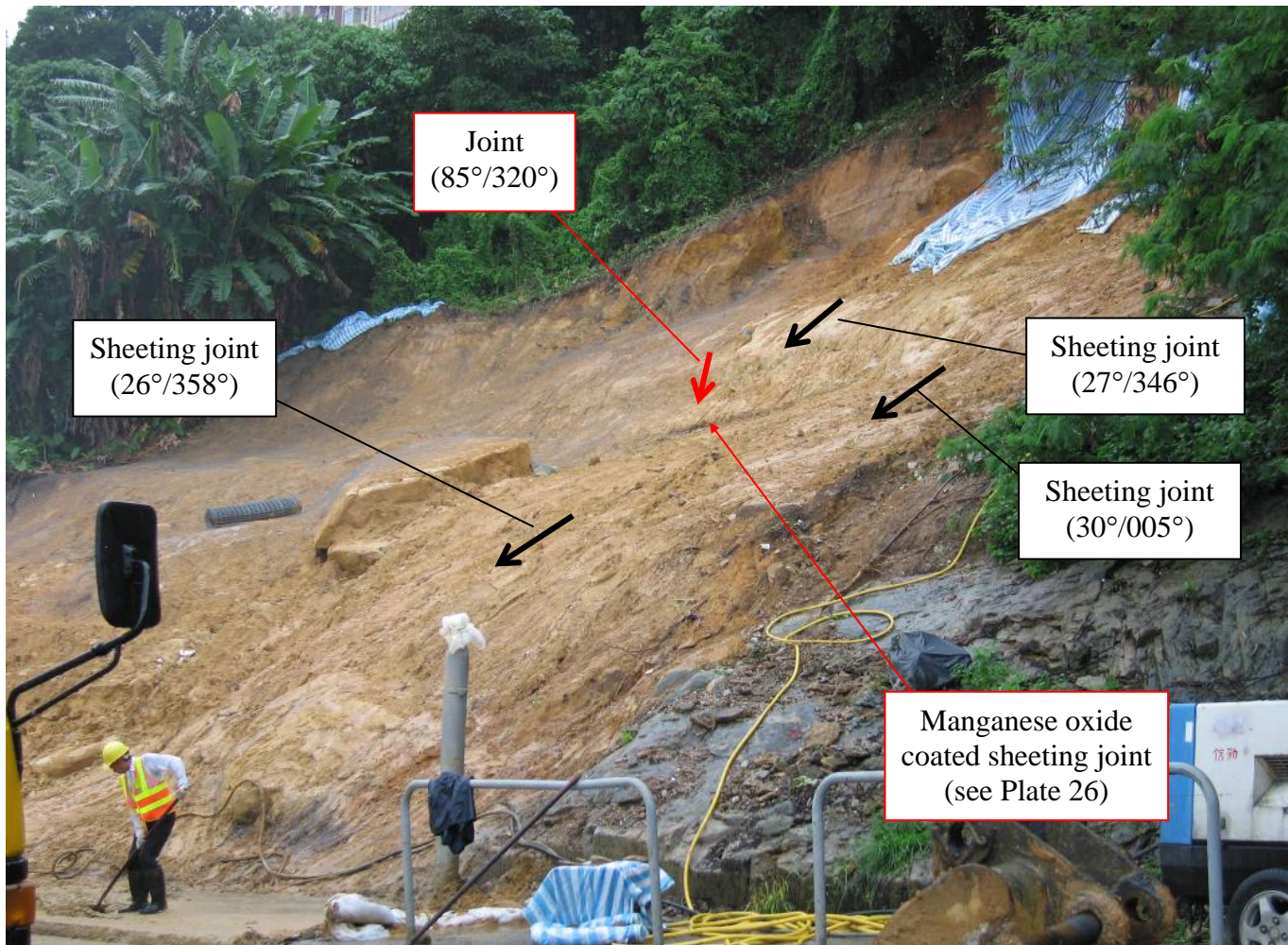
Plate 16 - Rupture Surface of the 7 June 2008 Landslide (Photograph taken on 18 June 2008)
