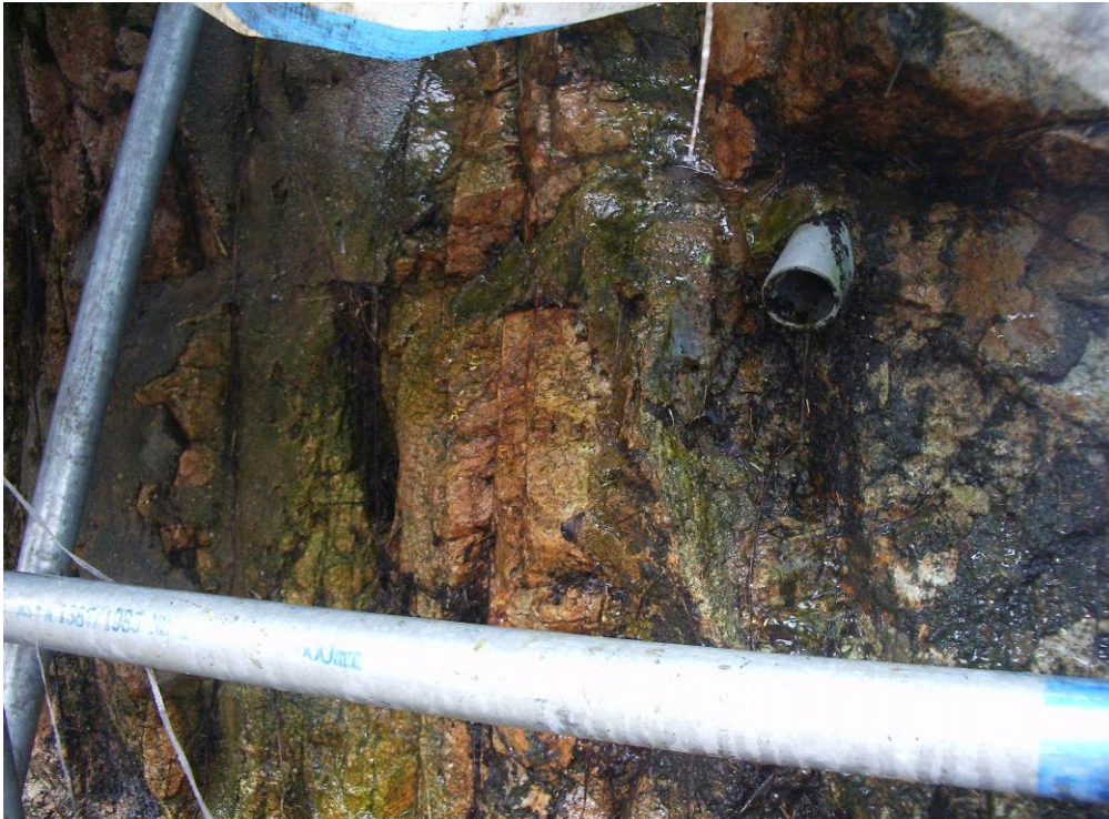
Plate 28 - Seepage at the Lower Portion of Slope No. 11SE-A/C710 (Photograph taken on 10 June 2008)
