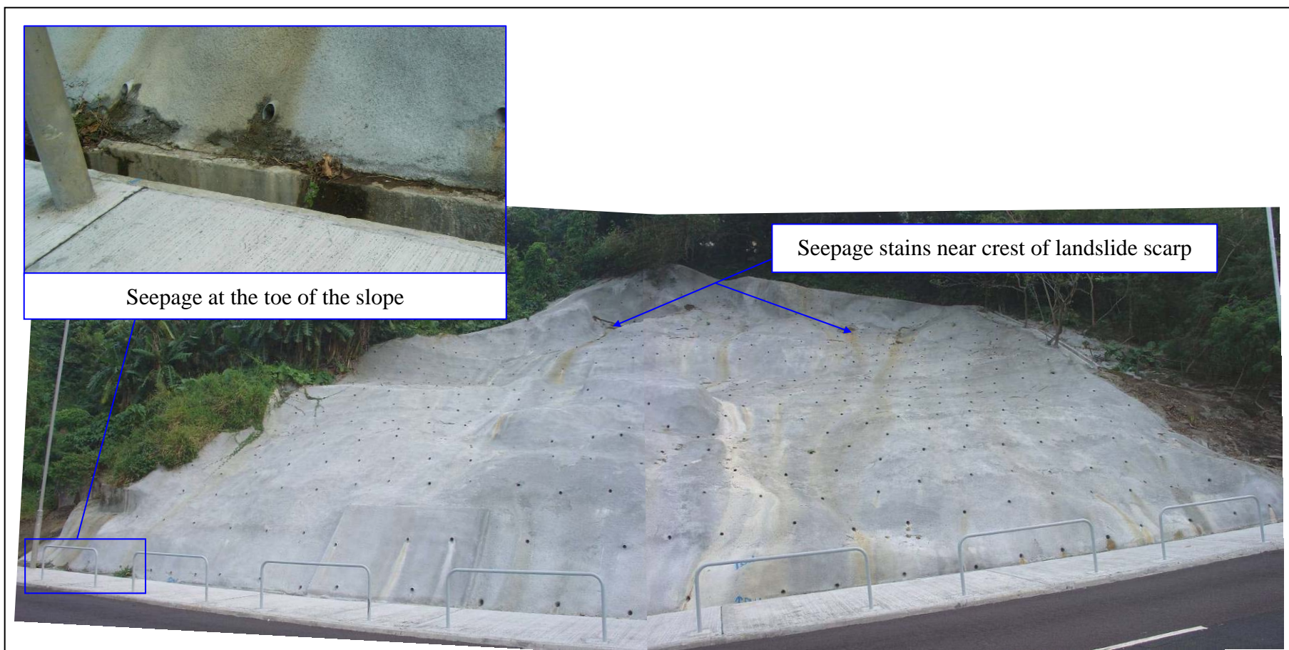
Plate 31 - Seepage Stains on the Shotcreted Landslide Scar (Photograph taken on 18 November 2008)
