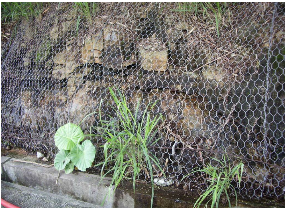
Plate 27 - Seepage from Toe of Western Portion of Slope No. 11SE-A/C502 (Photograph taken on 10 June 2008)
