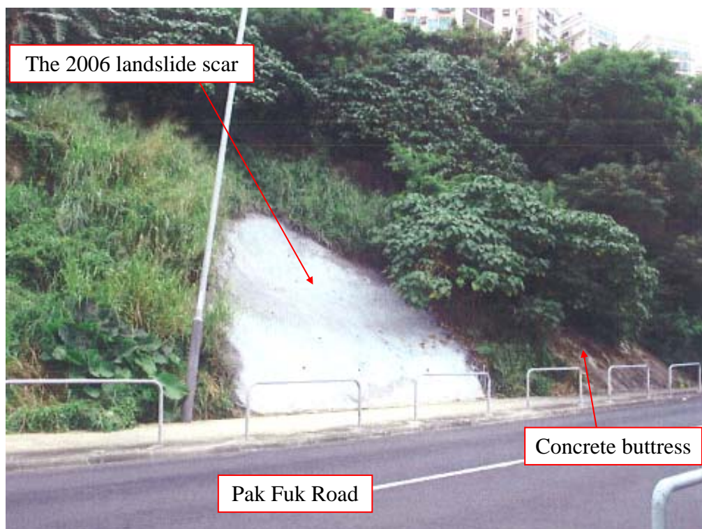
Plate 13 - The 2006 Landslide Scar after Completion of Emergency Repair Works (Photograph taken on 9 October 2006)
