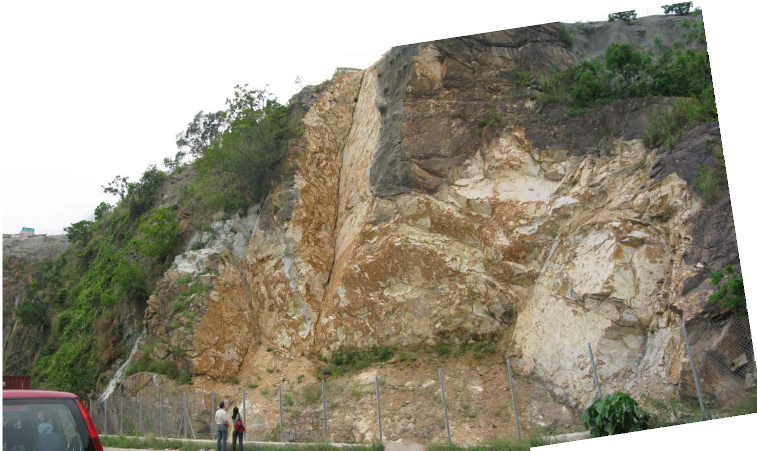
Plate 6 - General View of the Scar after Removal of Debris and Overhanging Rock Blocks (Photograph taken on 23 April 2009)
