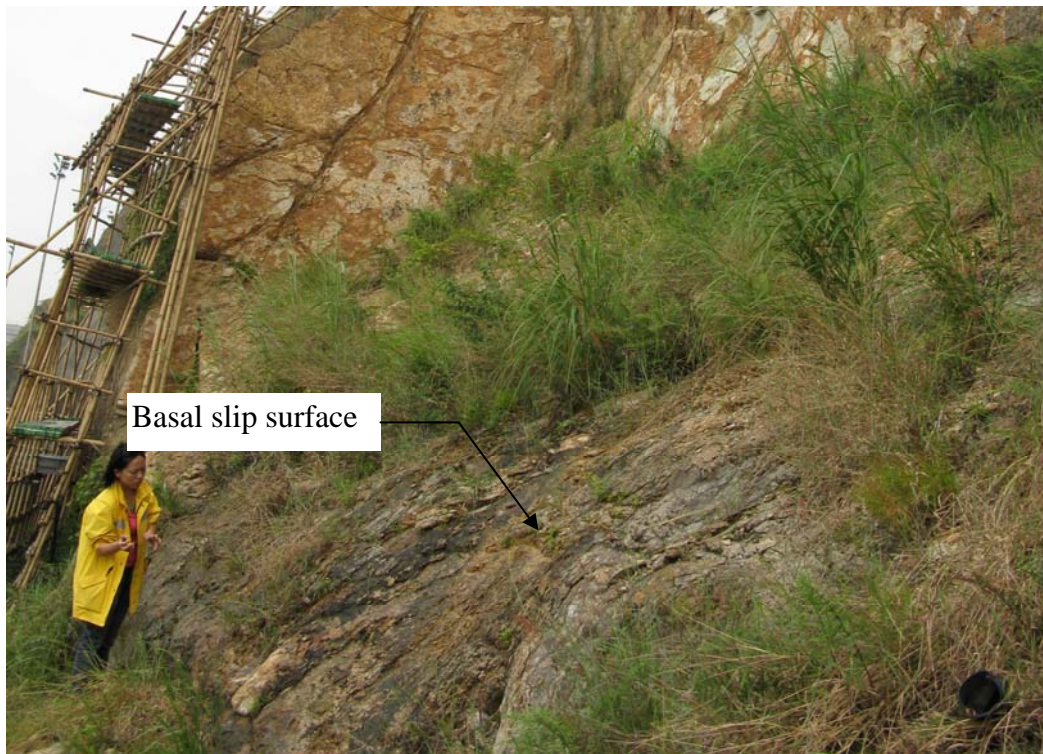
Plate 7 - General View of the Basal Slip Surface (Photograph taken on 20 October 2009)
