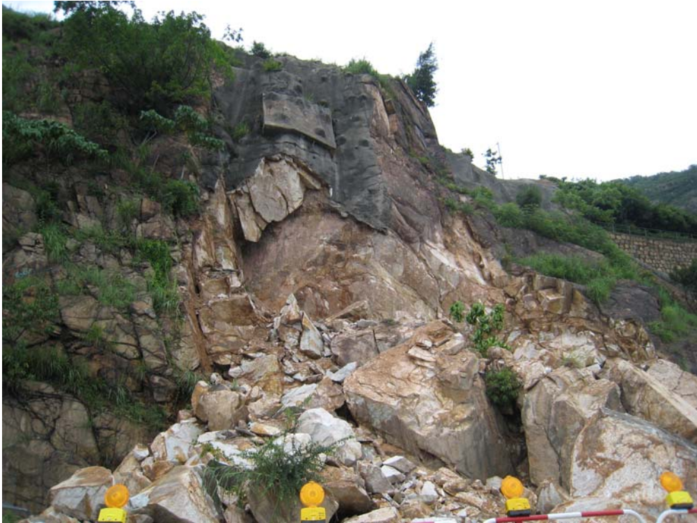
Plate 3 - Side View of the Rock Slope Failure towards the East (Photograph taken on 12 June 2008)
