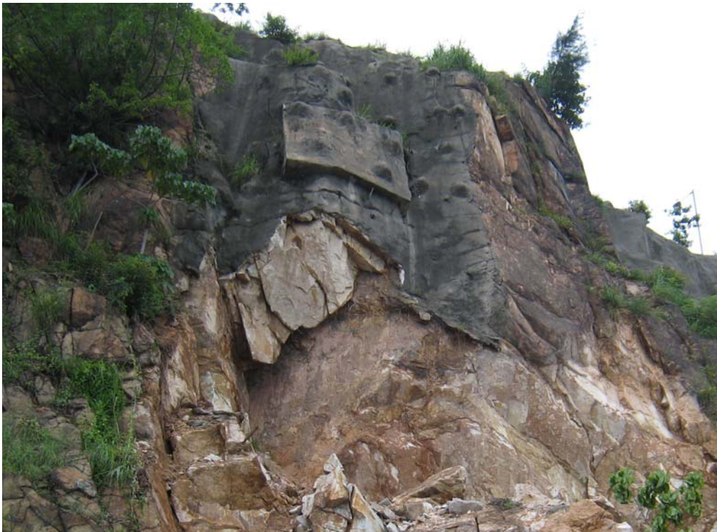
Plate 4 - Close View of Overhanging Blocks and the Rock Stabilisation Measures Installed in the 1980s above the Scar (Photograph taken on 12 June 2008)
