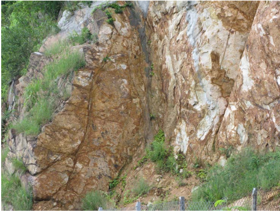
Plate 10 - Signs of Degradations and Heavy Staining at Release Joints (Photograph taken on 25 June 2009)
