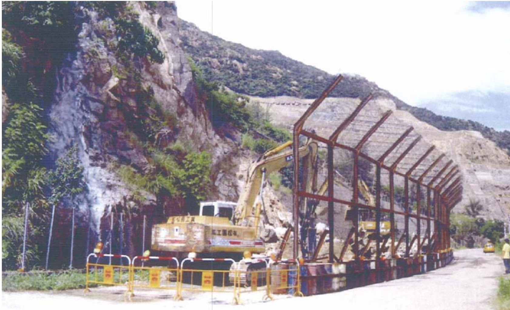
Plate 5 - Urgent Repair Works by the Highways Department after the 7 June 2008 Landslide
