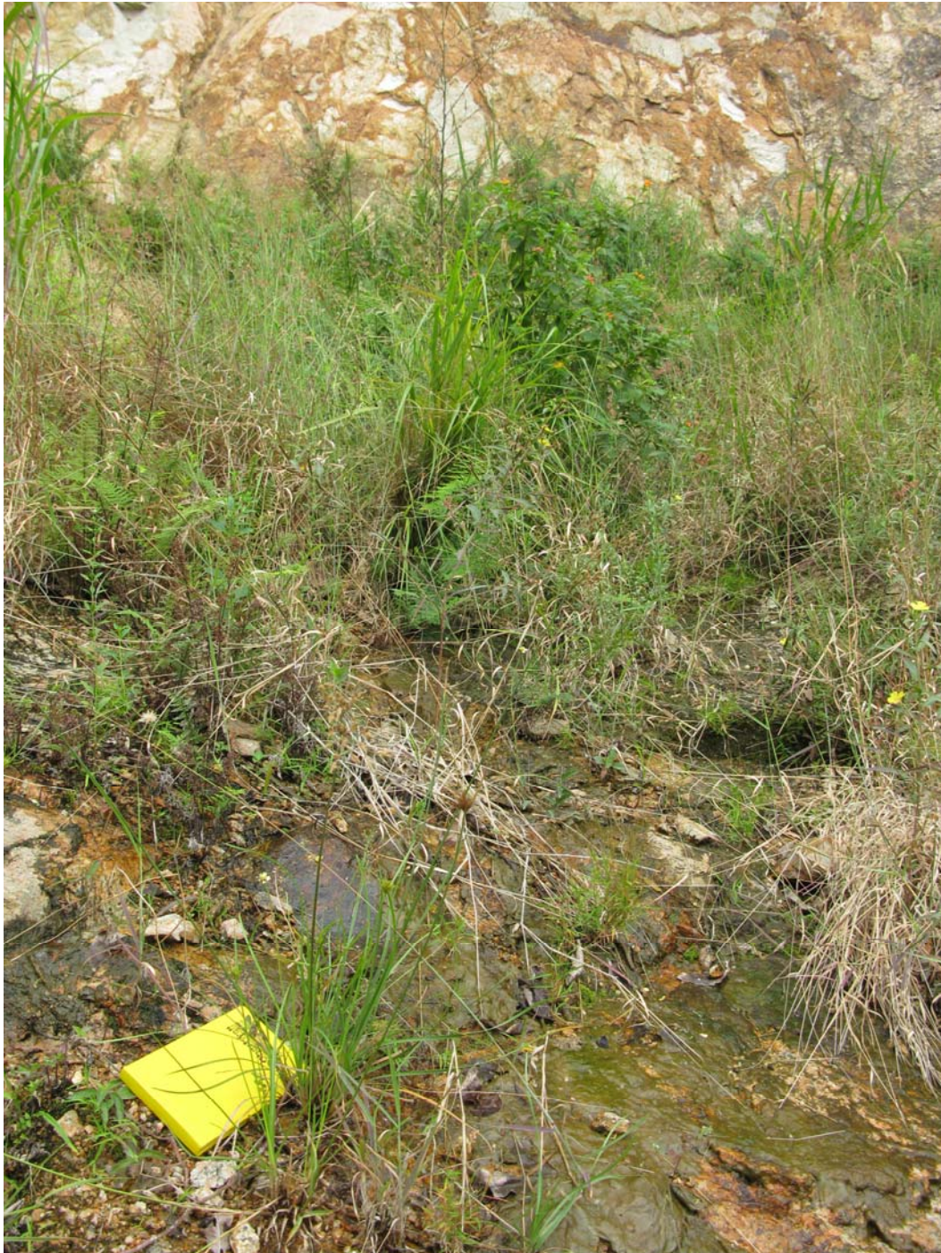
Plate 9 - Seepage with Growth of Algae Observed at the Basal Slip Surface (Photograph taken on 20 October 2009)
