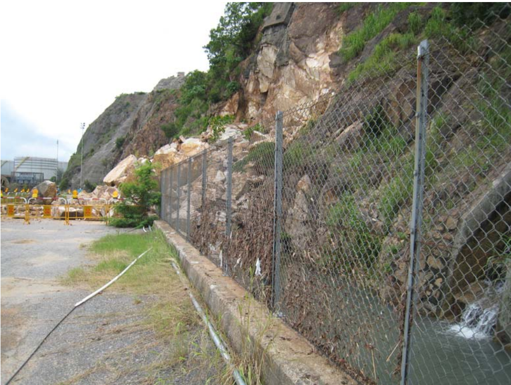
Plate 2 - Side View of the Rock Slope Failure towards the West and the Drainage Channel of Slope No. 10NE-B/C56 (Photograph taken on 12 June 2008)
