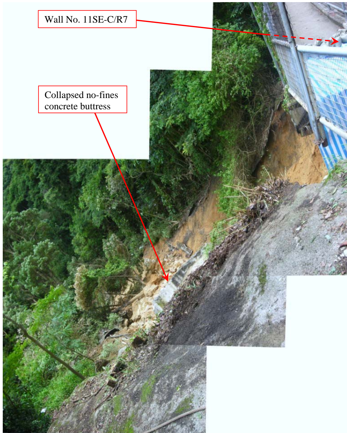
Plate 2 - Side View of the 30 June 2007 Landslide (Looking North) (Photograph taken on 30 June 2007)
