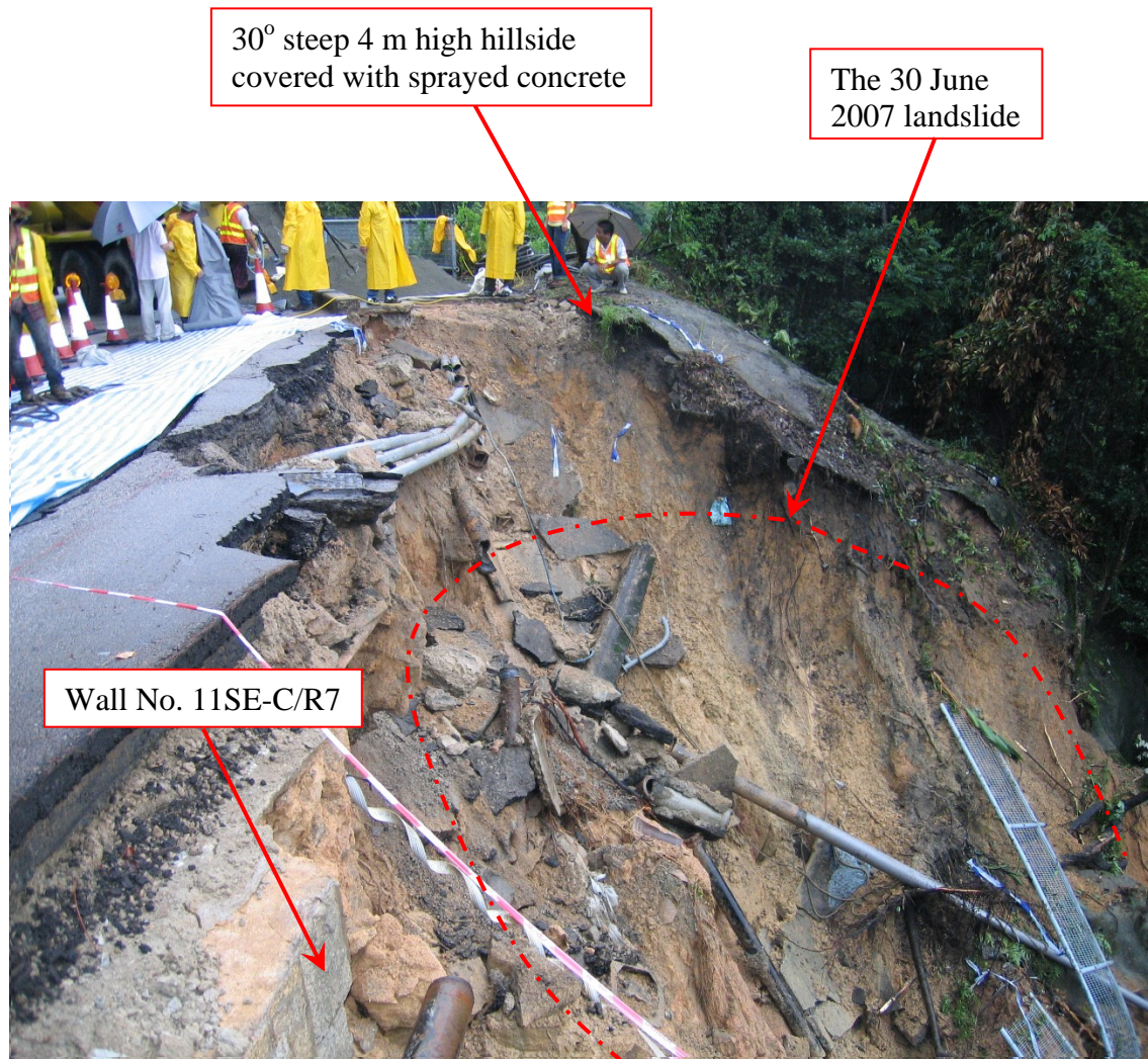
Plate 4 - Side View of the Upper Portion of the 30 June 2007 Landslide after Demolition of Elevated Pedestrian Pathway under HyD's Urgent Repair Works (Looking South) (Photograph taken by GEO on 30 June 2007)
