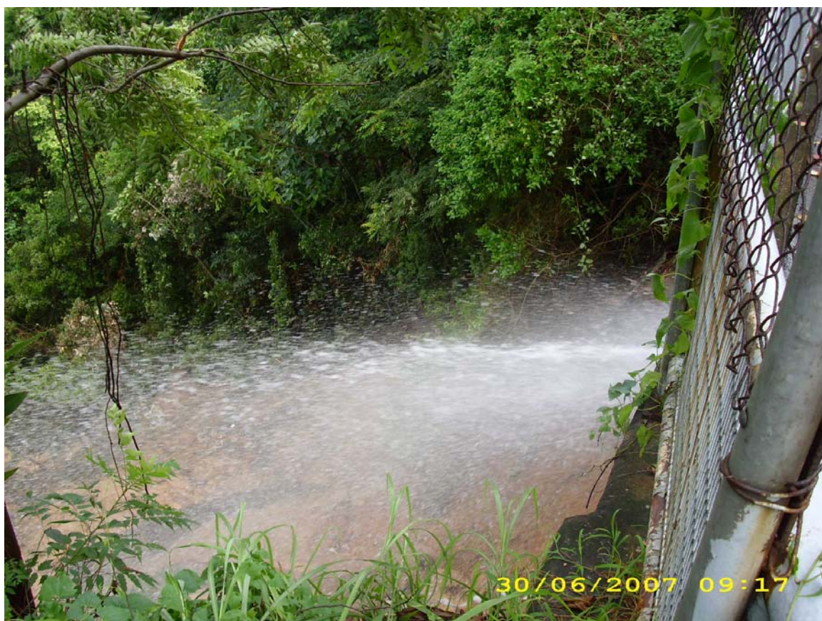
Plate 16 - Water Jet from the Burst Watermains (Photograph taken by Ove Arup & Partners Hong Kong Ltd.on 30 June 2007)
