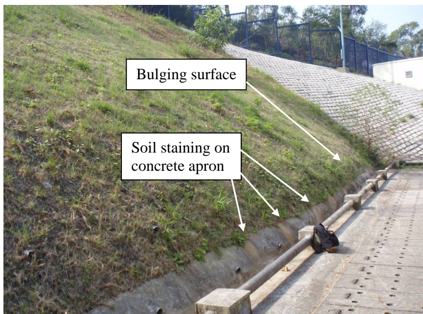
Plate 12 - Soil Staining and Bulging Observed at the Toe of Slope No. 3SW-C/C234 (Photograph taken by HCL on 18 December 2007)
