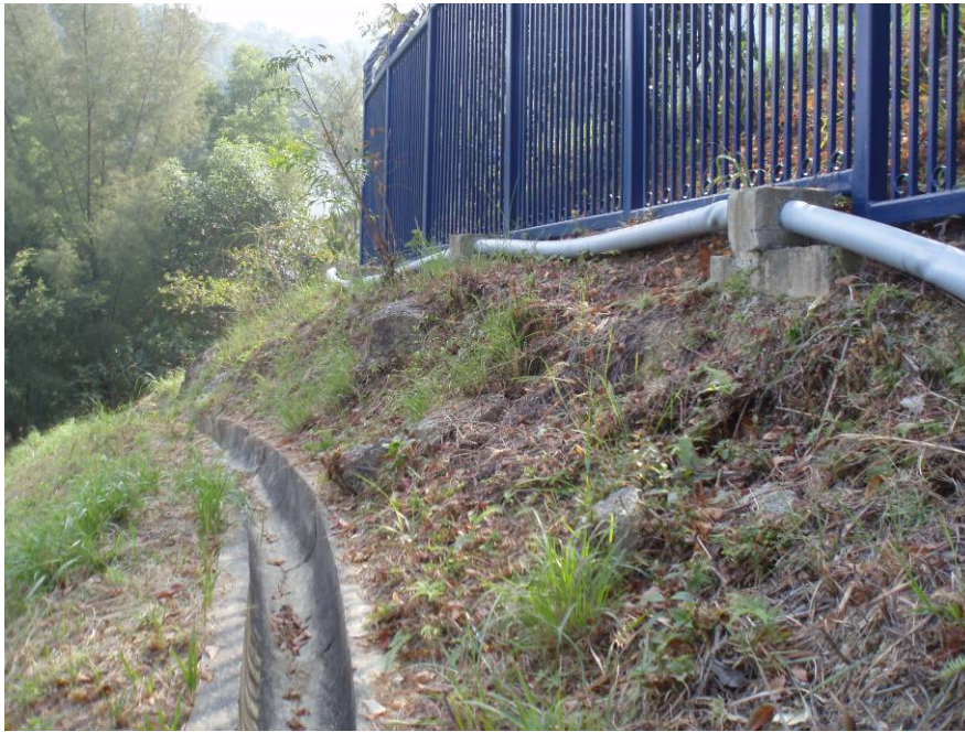
Plate 7 - A 100 mm Diameter PVC Pipe Running along the Crest of Slope No. 3SW-C/C234 (Photograph taken by HCL on 18 December 2007)
